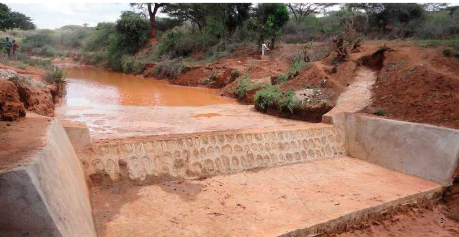
Figure 1-1 Example of a sand dam
