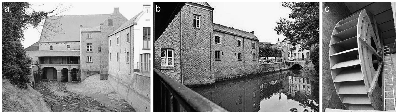
Figure 2. (a) So-called Spanish mill, dating from the 16th century, only remaining tide mill in Flanders (Rupelmonde, Province of East Flanders, Belgium). (b) Retention basin of the tide mill (restored) (c) New 6 m diameter tide mill wheel. Photographs owned by and reproduced courtesy of Official Tourism Office of the city of Rupelmonde-Bazel-Kruibeke.
