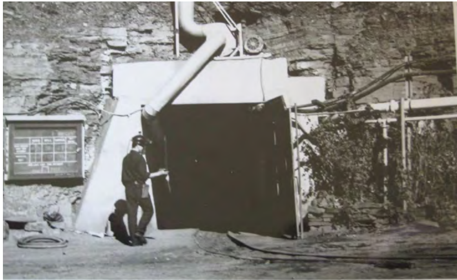
Figure 26: The entrance (adit) to the mine c. 1957. Photo courtesy Sue Ranieri.
