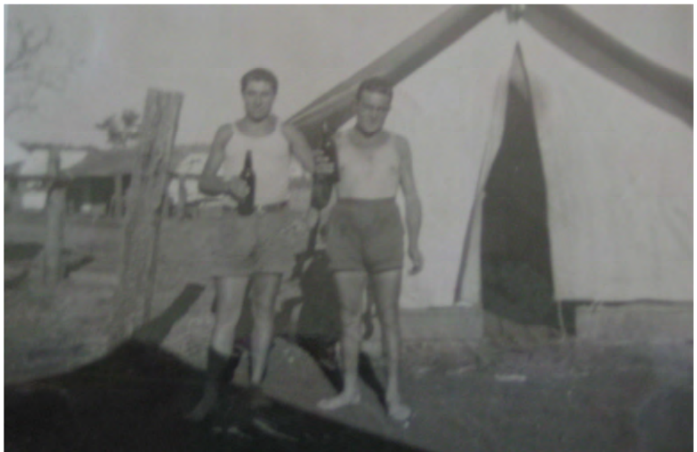
Figure 45: Single men's accommodation. Photo courtesy Sue Ranieri.
