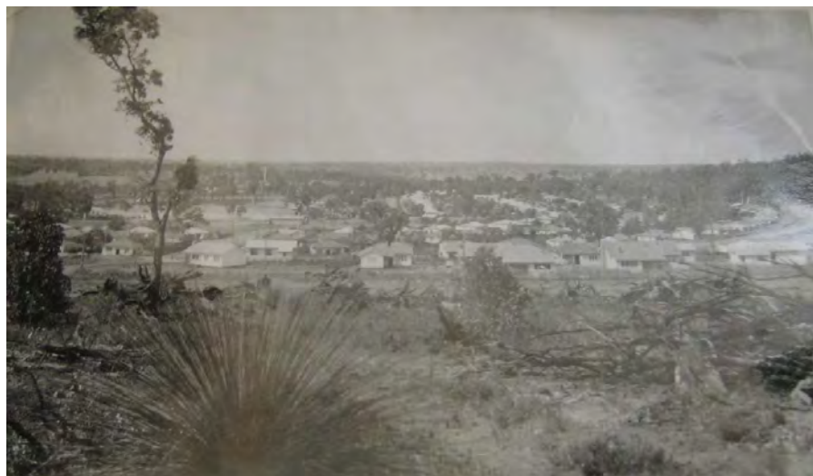
Figure 18: Wundowie's asbestos houses. Photo courtesy Pio Panizza.
