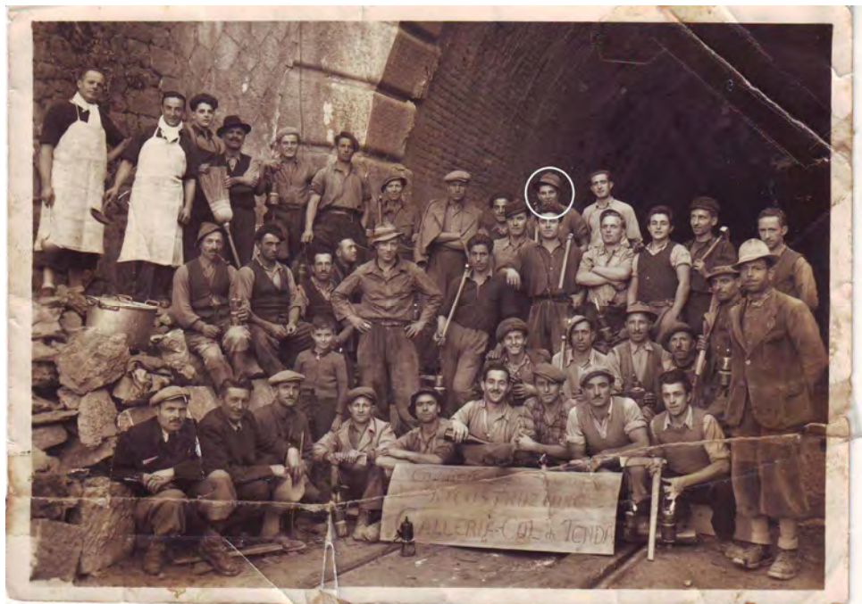
Figure 12: Attilio Oprandi at the Alpine tunnel construction site of the Galleria Col di Tenda, Piedmont, linking Italy and France. Photo courtesy Frank Oprandi.
