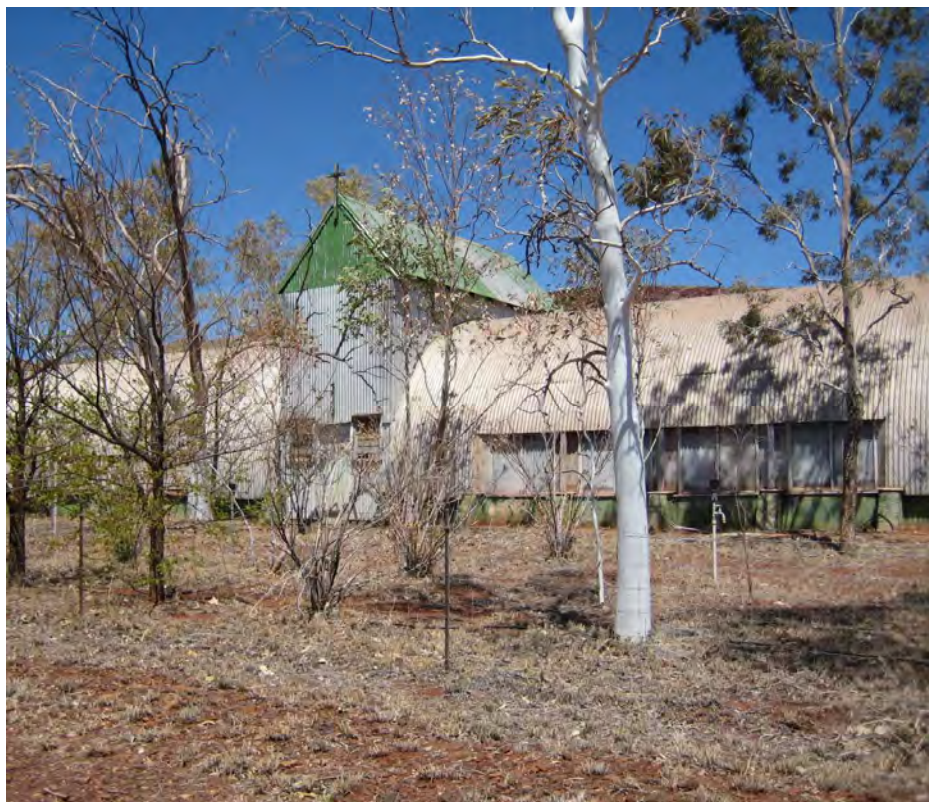
Figure 81: Wittenoom Catholic church one of the few remaining buildings in September 2010.
