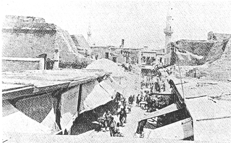
Fig. 12 Chania at the beginning of 20 th century. The demolition of the southern walls and of Porta Rethimniota.
