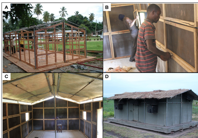
Figure 3: Ifakara experimental huts. Panel A shows the main framework of the huts under construction at the workshop. Panel B shows technicians fitting the wall panels, (made of chicken wire on wooden frames), onto the inside walls of the huts. Panel C shows the inside surfaces of the huts after fitting the wall panels and also the palm woven ( mikeka ) ceiling on the underside of the steel roof, but before the inside walls are covered with mud, and Panel D shows a completed and functional Ifakara experimental hut, fitted with interception traps on windows and eave spaces and thatched over the steel roof with grass to match indoor temperatures of local dwellings. The overall shape and dimensions are those of typical local houses. The hut is suspended on water-filled metal bowls to prevent predator ants, which would otherwise prey on the trapped or dead mosquitoes in the huts.
