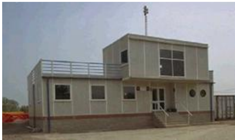
Figure 2.12. Severn Crossing road bridge site office and later visitor information centre constructed with the ACCS (courtesy of Sharon Loxton).
