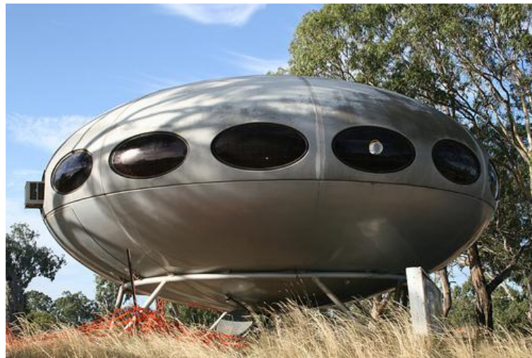
Figure 2.9. Weekend chalet of 36 GRP sections of double-skinned sandwich construction (via http://www.worldarchitecturemap.org ).
