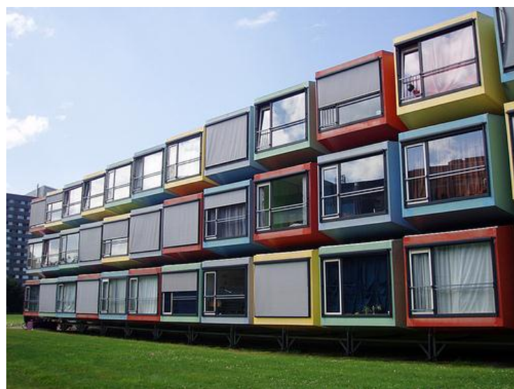
Figure 2.10. The SpaceBox volumetric and modular system (courtesy of www.spacebox.nl )
