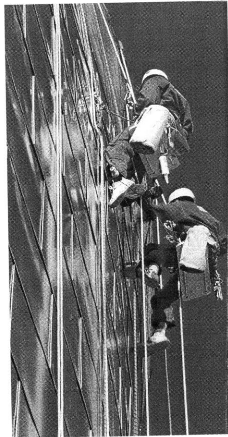
Figure 8 – Workers installing titanium cladding
