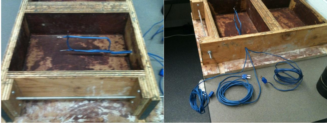
Figure 2. Thermocouples prior to concrete placement
