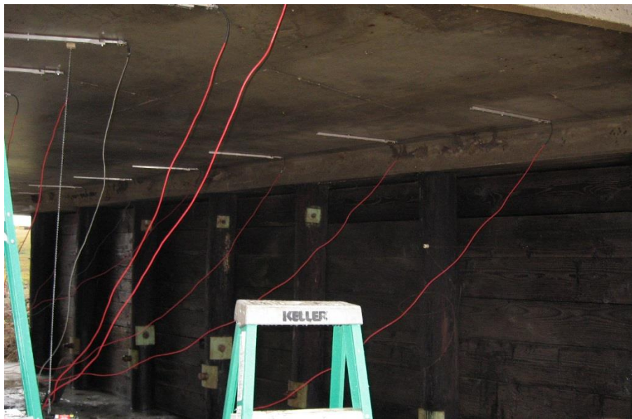
Figure 11. Johnson County Bridge instrumentation setup
