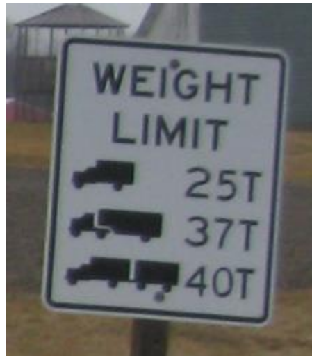
Figure 4. Johnson County Bridge load posting
