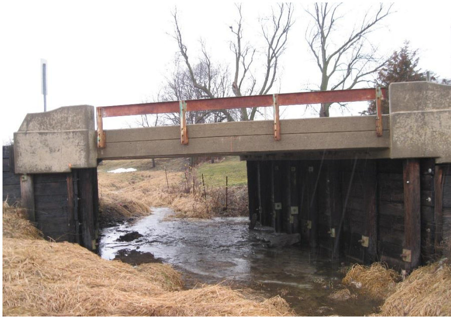
Figure 3. Johnson County Bridge elevation view
