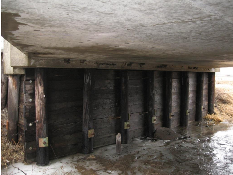
Figure 5. Johnson County Bridge bearing
