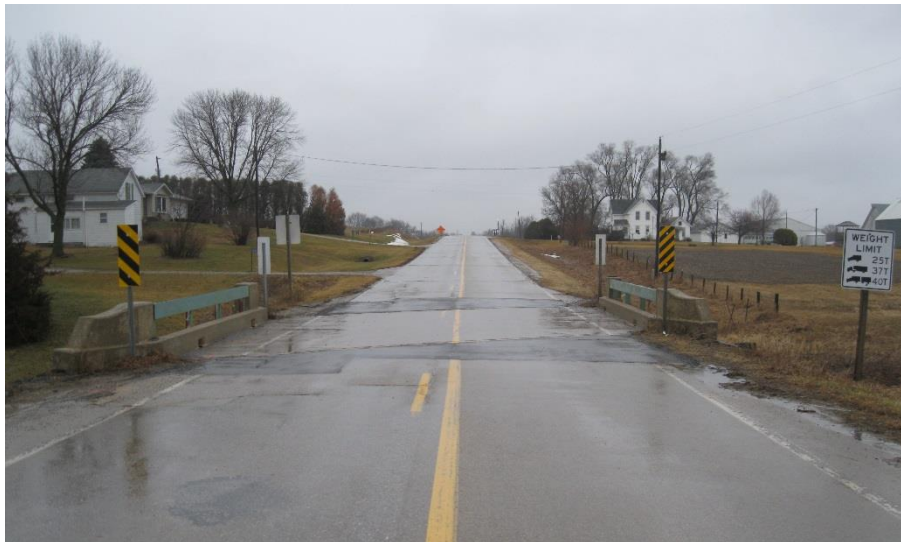
Figure 2. Johnson County Bridge end view
