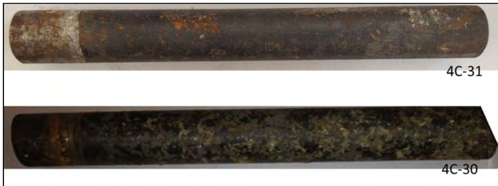
Figure 4-19 Active steel bars of sample 4C-31 and 4C-30, just after taken out from concrete
