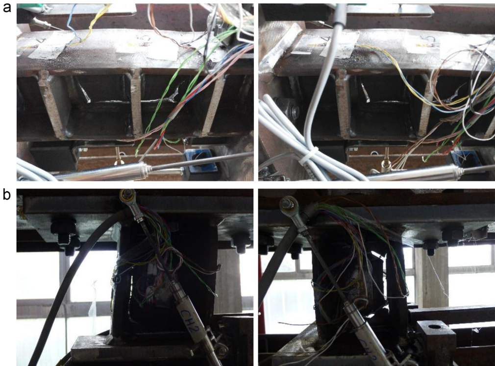
Fig. 10. Progressive damage in the (a) horizontal and (b) vertical links due to the execution of experimental tests.
