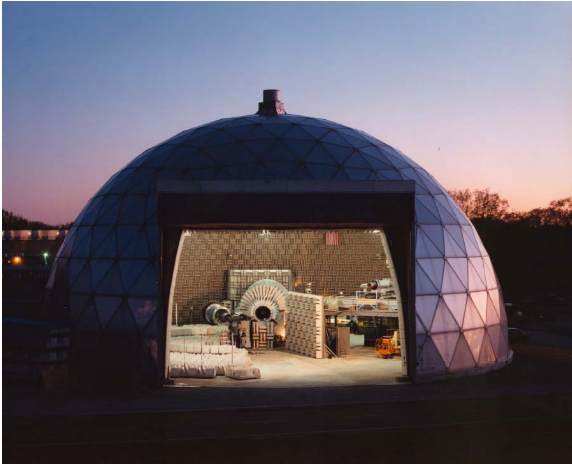
Figure 1. Aero-Acoustic Propulsion Laboratory
