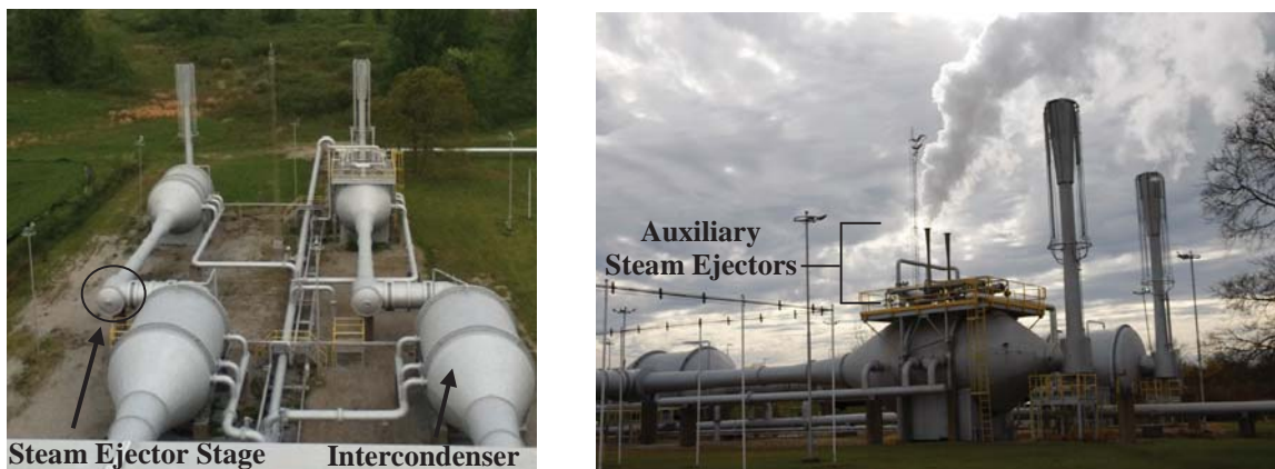
Figure 3. ISP Facility steam ejectors. (Left) Main steam ejectors used in baseline altitude propulsion testing. Typical steam ejector stage and intercondenser highlighted. (Right) Auxiliary steam ejectors shown exhausting steam on top of the east second stage intercondenser.
