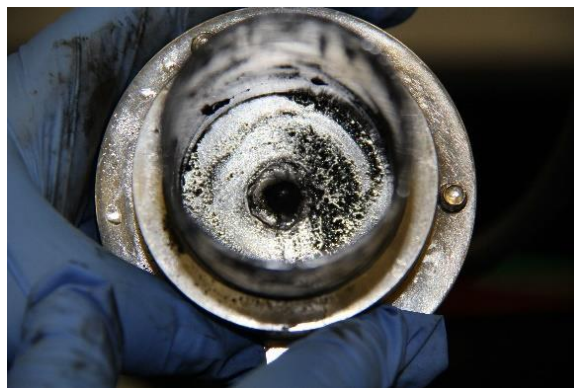
Figure 6. Carbon plugging the outlet endcap.
