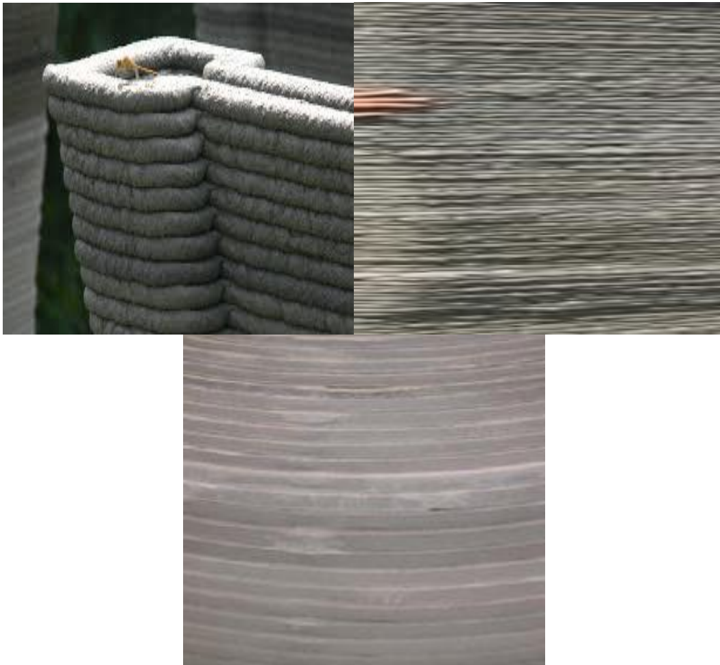
Fig. 2 Surface finish of (a, b) typical concrete deposition and (c) Contour Crafting deposition
