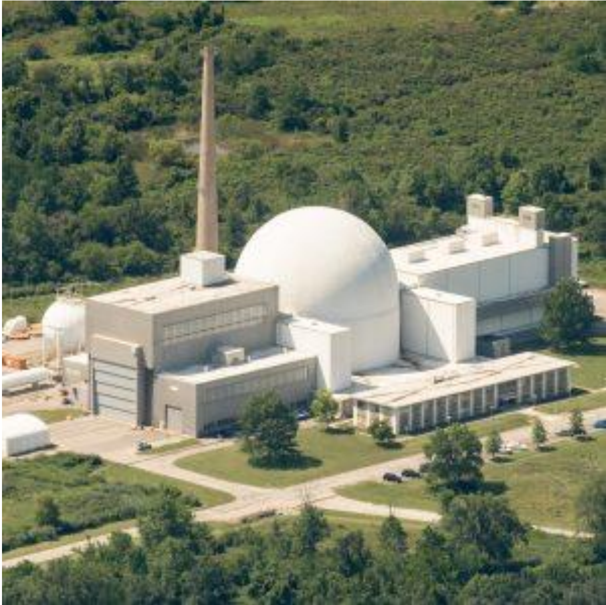
Figure 9: Space Environments Complex (SEC) aerial view.
