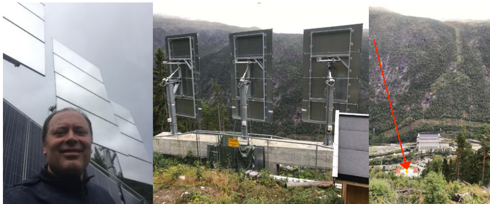
Figure 1.7. Top row: Heliostats illuminating towns in deep valley at Rjukan, Norway. Bottom row: NIAC Fellow Stoica, after a hike at Rjukan, next to the mirrors; back of mirrors and location where sunrays are redirected in town plaza, at ~700 m away from the mirrors.
