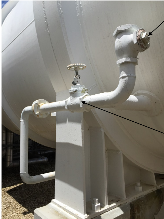
VACUUM PIPING WITH VALVE AND SAFETY DEVICE
