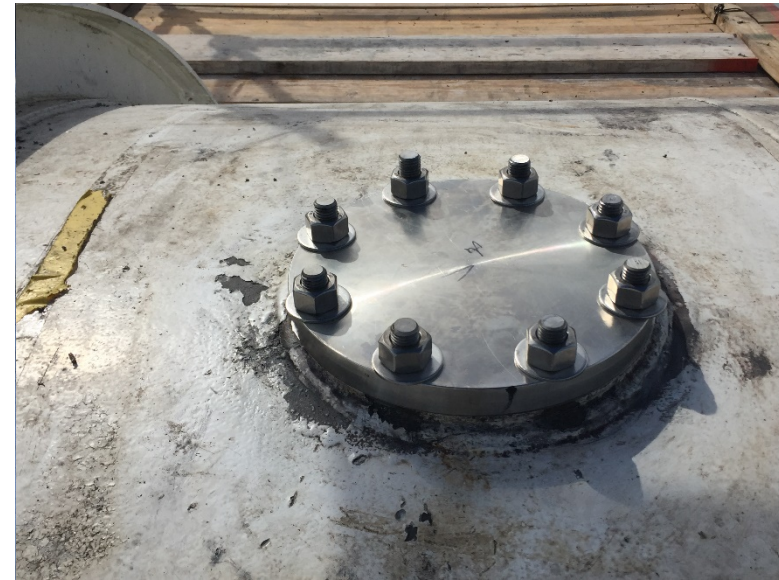
32 RMS finish with 316 S.S Studs and blank flange with O-ring groove and Viton O-ring(AS568)
