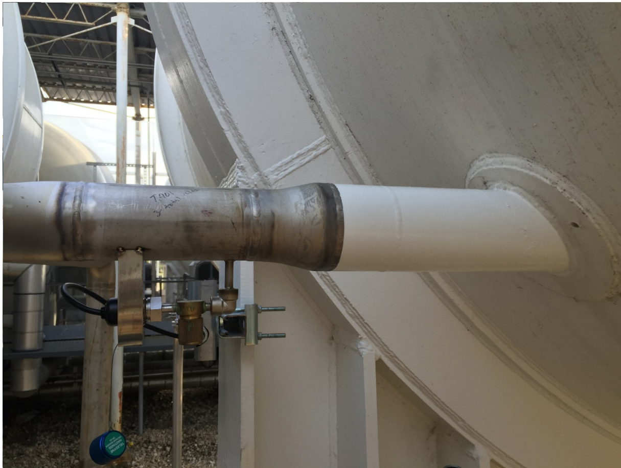
NEW INSTALLED PIPING WITH COATING
