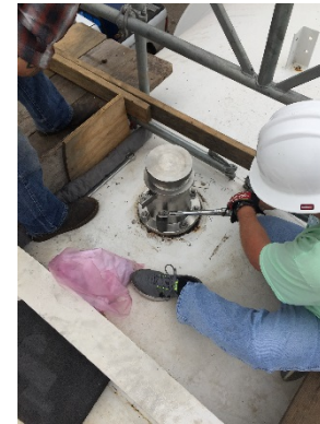
New Safeties Installed
