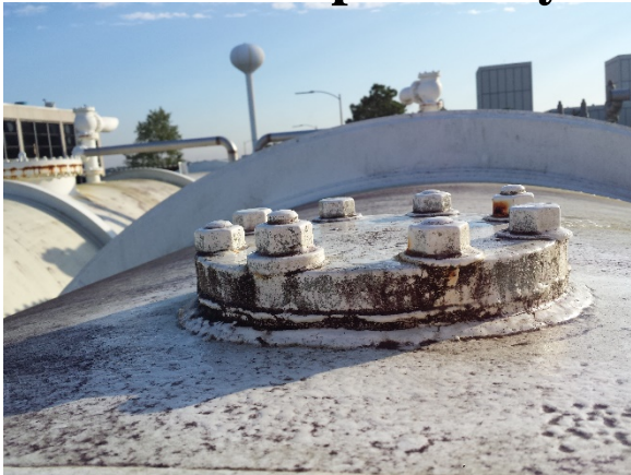
Pearlite Fill Flange, Carbon Steel
