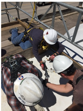
Removing Existing Flanges
