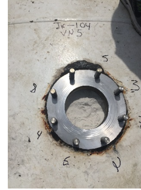
Final with New S.S. Studs
