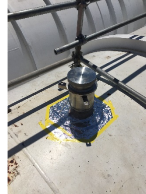
Completed Welded Assy
