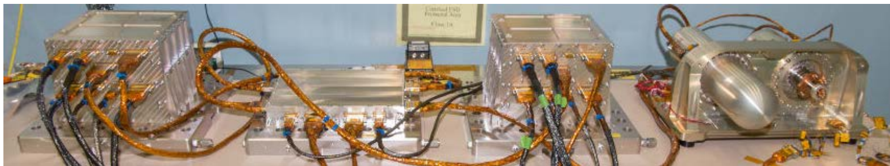
Flight Cyocooler Control Electronics, Redundancy Switch Electronics, and Thermal Mechanical Unit at GSFC
