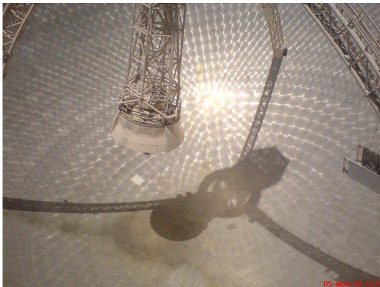
Figure V.A.3: View of 54m diameter spherical primary reflector of millimeter-wavelength radio telescope in Armenia. The on-axis corrector is seen mounted at the end of a pivot arm supported by a tripod structure.
