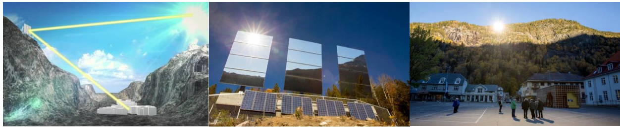
Figure 1.3. Heliostats illuminating towns in deep valleys: Rjukan (Norway) and Viganella (Italy). SOURCE: http://sourceable.net/century-old-engineering-idea-brings-sun-to-mountain-town
