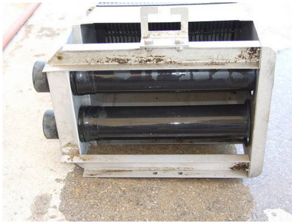
Figure 3.14 MBR3: Air diffusers
