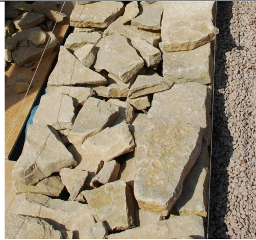
b) Wall 3 Construction
