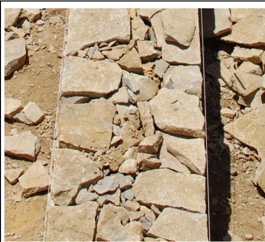
a) Wall 1 Construction
