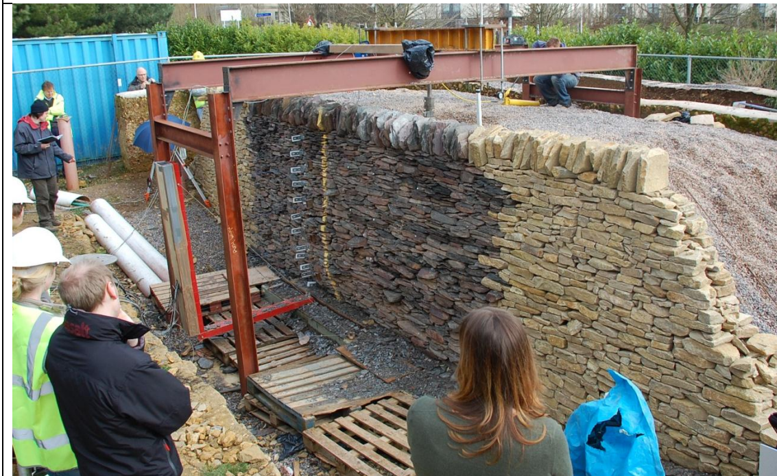
a) Schematic cross-section through a test wall, and (b) overview of Wall 5 during testing.
