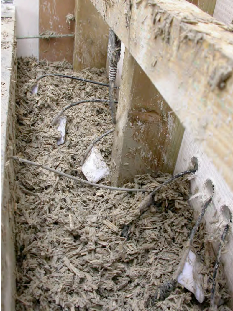
Figure 3: Sensors embedded in the hemp-lime wall during construction
