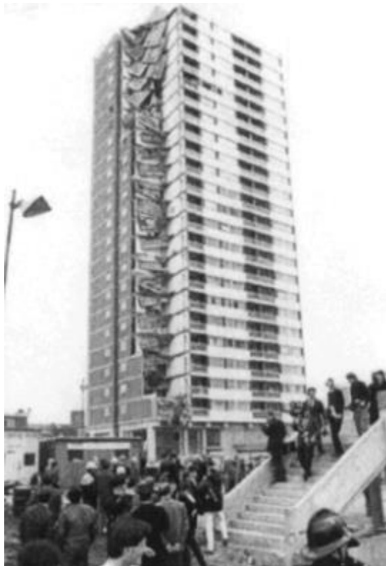
Figure 2-1 Disproportionate collapse at Ronan point apartments in London England (Osama 2006)
