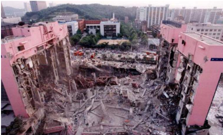
Figure 2-2 North wing collapse of Sampoong Department Store
