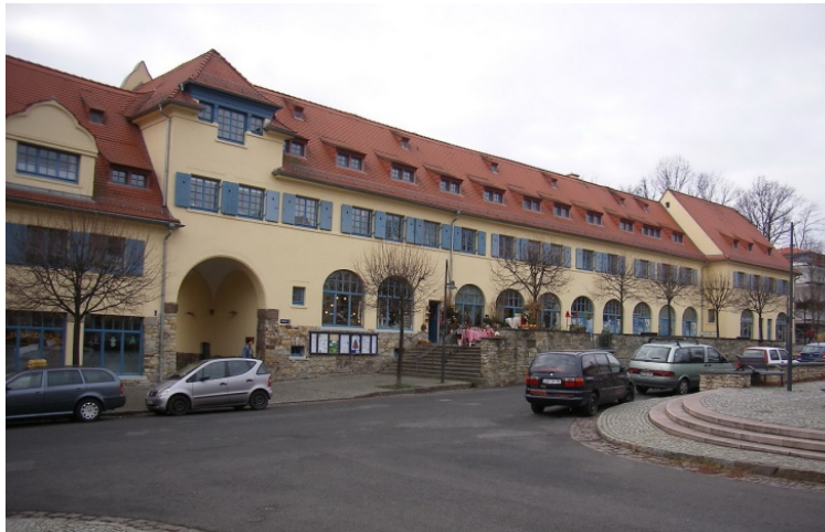
Figure 102. Richard Riemerschmid, market building, Gartenstadt Hellerau, ca. 1910.
