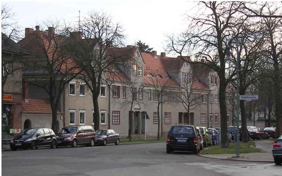
Figure 73. Paul Schmitthenner, apartment buildings, Am Heideberg, Gartenstadt Staaken, ca. 1914.
