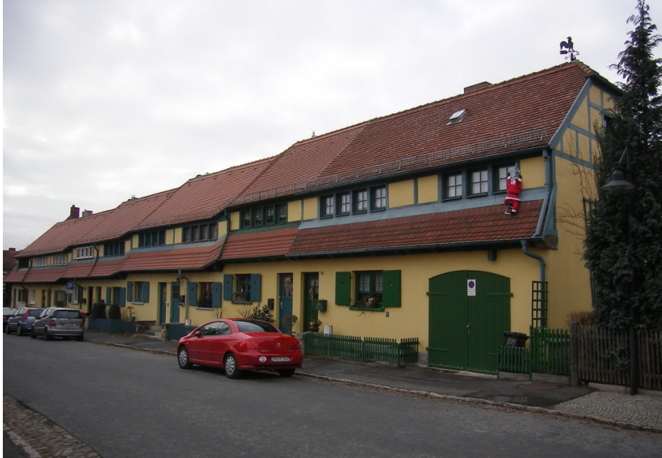
Figure 26. Richard Riemerschmid, row houses along Am Grünen Zipfel, Gartenstadt Hellerau, ca. 1909. Riemerschmid used the change in elevation as aesthetic inspiration, allowing the roofline of the houses to step down the incline of the street. A downward pointing arrow marks this street on Figure 23.
