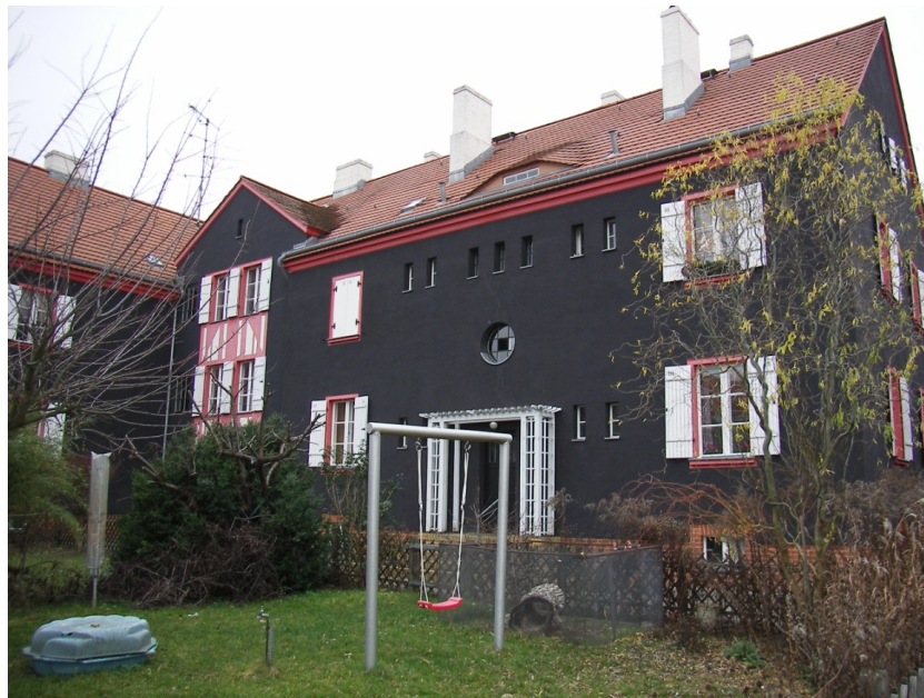
Figure 91. Bruno Taut, apartment building on Gartenstadtweg, Gartenstadt Falkenberg, ca. 1914. The black façade, with contrasting painted decoration, reveals Taut's dramatic use of color. The dark color also allowed Taut to manipulate the viewer's spatial impression of the street.
