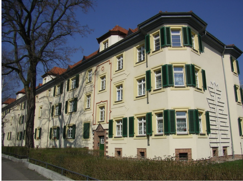
Figure 86. Apartment building, corner of Triftweg and Lerchenrain, Gartenstadt Marienbrunn, 1928. The brick at the foundation and around the doors and cellar windows emphasized the base of the building and revealed the underlying structure just as Taut had done at Gartenstadt-Kolonie Reform, although in a much more decorative fashion.
