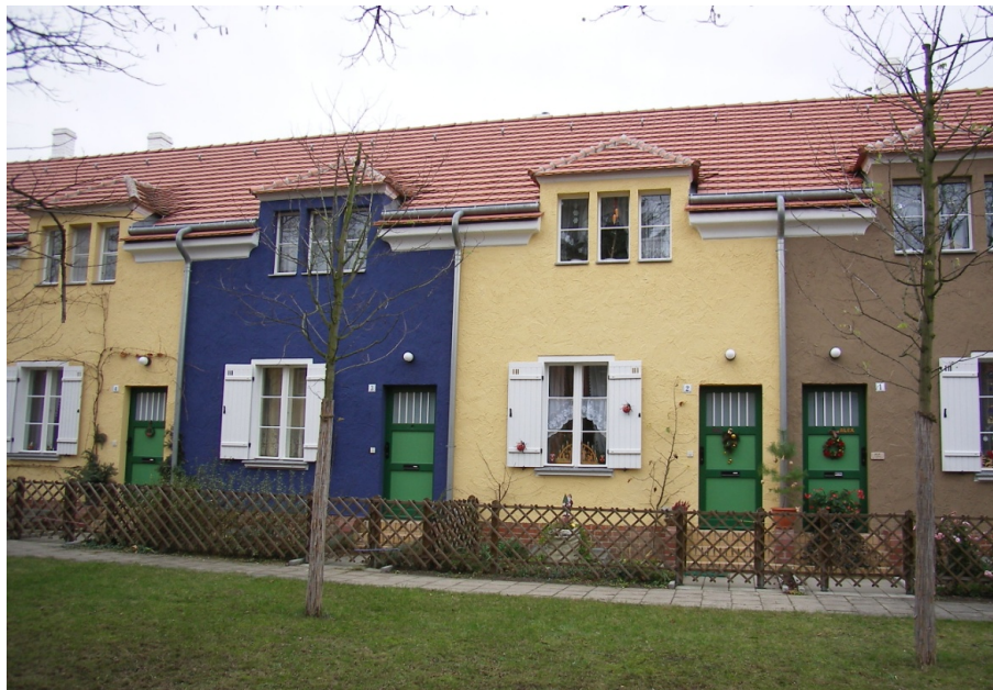
Figure 93. Bruno Taut, row houses, Akazienhof, Gartenstadt Falkenberg, ca. 1913. The houses are painted the bright colors associated with Taut. While their façades are not purely symmetrical, Taut maintains a sense of balance and rhythm.
