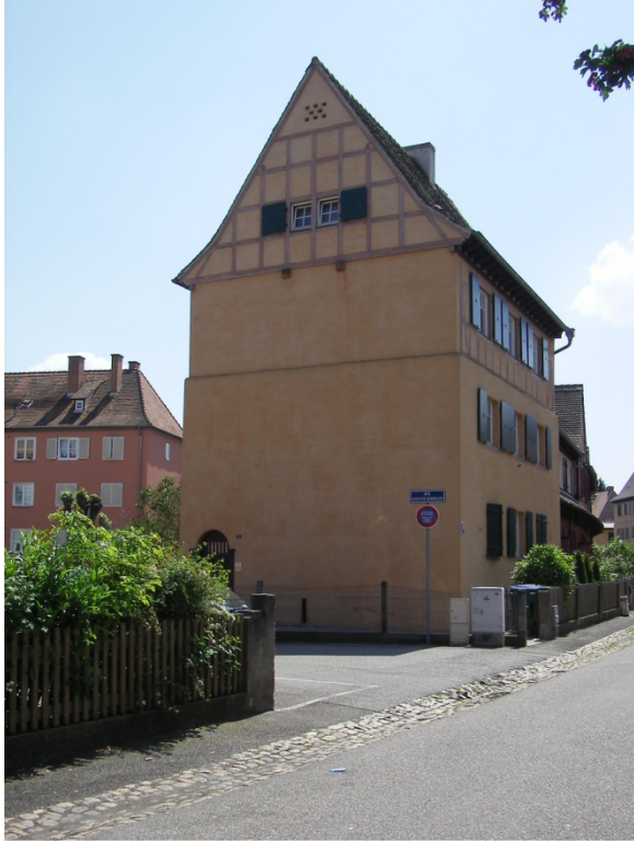
Figure 88. Multi-family residence, Gartenstadt Stockfeld, ca. 1911. The half-timbering here appeared much more traditional than Tessenow's version below due to the steeply pitched roof, despite the fact that both utilized simple grid patterns.
