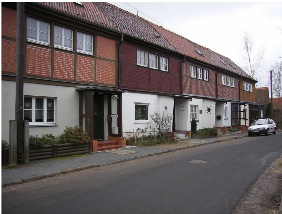
Figure 89. Heinrich Tessenow, row houses, Am Pfarrlehn, Gartenstadt Hellerau, ca. 1912. The exposed brick is a reinterpretation of the traditional half-timber building technique.
