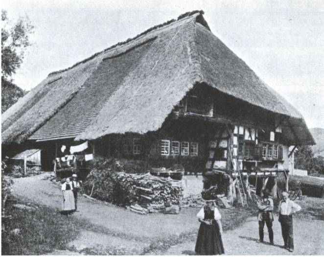
Figure 81. Farmhouse in Baden. The proportion of roof to wall is typical of many vernacular buildings, as is the half-timbered wall construction.
