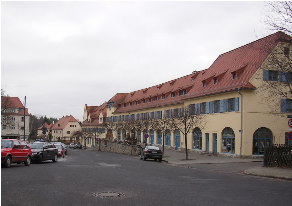
Figure 27. Richard Riemerschmid, Marktplatz, Gartenstadt Hellerau, ca. 1910. By establishing a stone plinth at the base of the building, Riemerschmid was able to create a flat terrace in front of the shop arcade.
