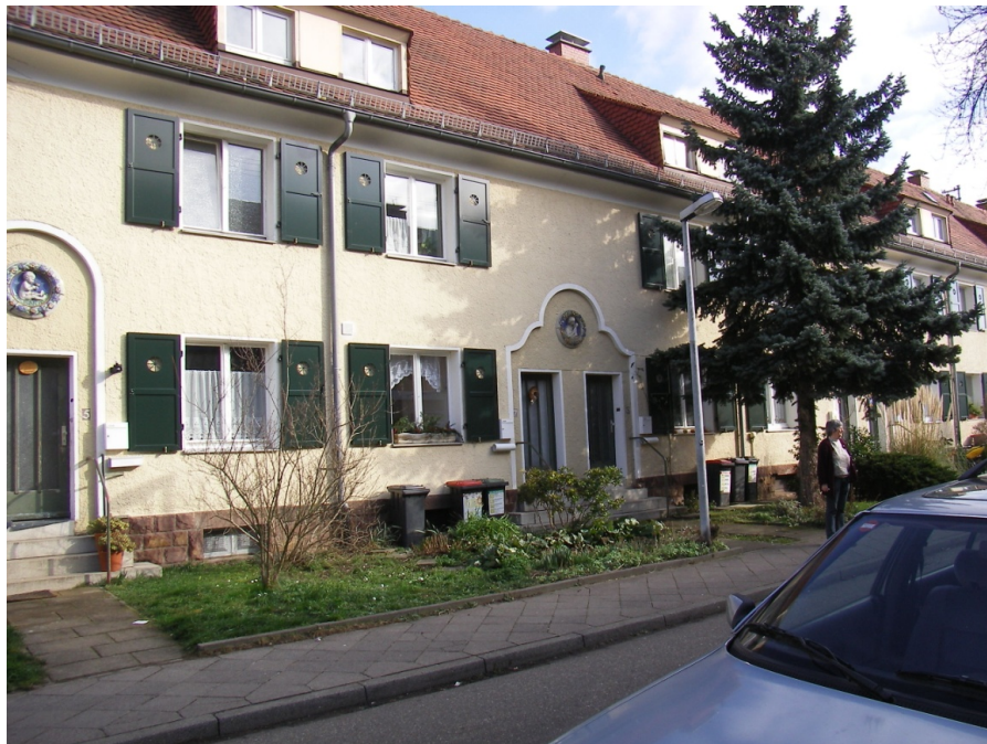
Figure 87. Row houses, Gartenstadt Karlsruhe, ca. 1910-11. Applied molding around the doors enlivened an otherwise completely flat façade.
