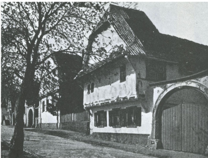
Figure 83. Farmhouse from the Rheinpfalz. Riemerschmid used the small roof projecting from the façade on his row houses at Hellerau (ca. 1909). See Figure 26.
