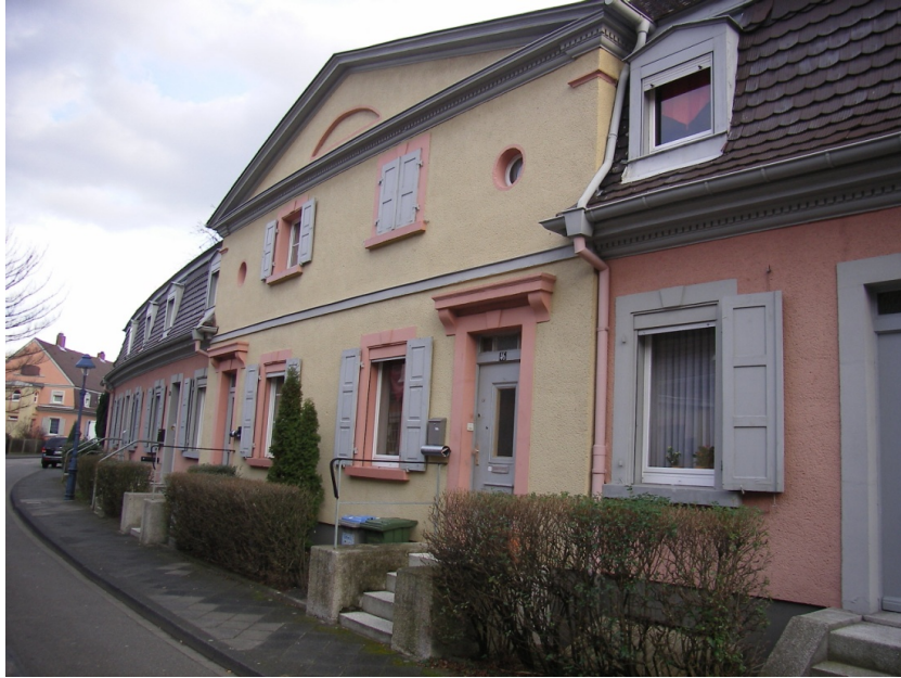
Figure 92. Esch & Anke, row houses, Westring, Gartenstadt Mannheim, ca. 1914. The classical detailing is one of the few instances of applied decoration in the garden cities. Notice also the symmetry of the central pavilion. It is unclear from the available sources whether the color of the stucco was original.
