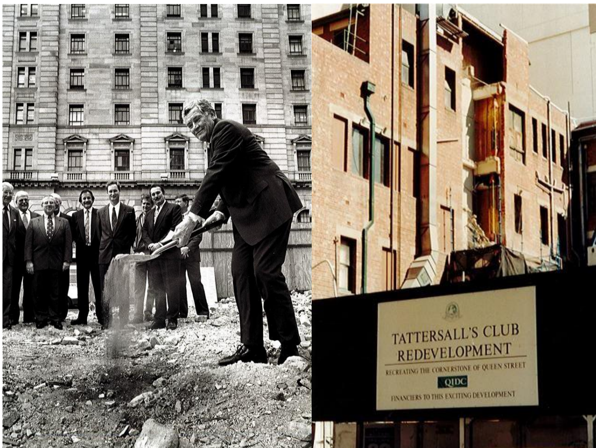
Fig. 46. (left) Tattersall’s President John O’Duffy ‘turning the first sod’ on 4 August 1995; (right) the vacant corner site as construction begins. (Photos: Tattersall’s Club archives).
