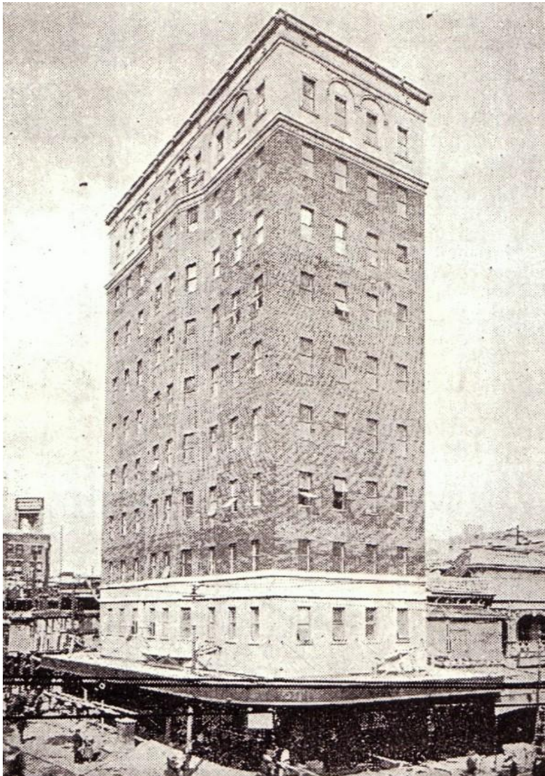
Fig. 44. Ascot Chambers on the corner of Edward and Queen Streets, photographed shortly after its completion in 1925. At the time, the original Tattersall’s building on Edward Street was still being constructed to the left of Ascot Chambers. The proposed extensions in the 1990s would occupy the entire corner site. (Photo: Brisbane Courier , 25 August 1925).
