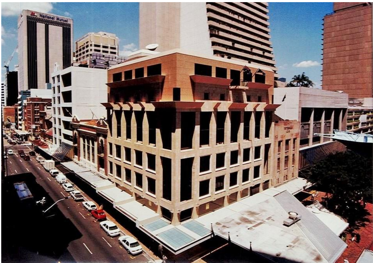
Fig. 47. The new Tattersall's building. In adjoining the Club's 1926 Edward Street property (to the left), and its 1939 Queen Street property (to the right), the new structure consolidated Tattersall's premises across the entire corner of Edward and Queen Streets. (Photo: Rene Marcel, 1997).
