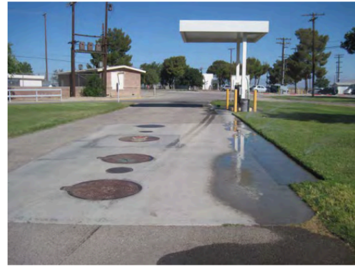
Fuel station with one 4,000-gallon diesel fuel UST and one 8,000-gallon gasoline UST.
