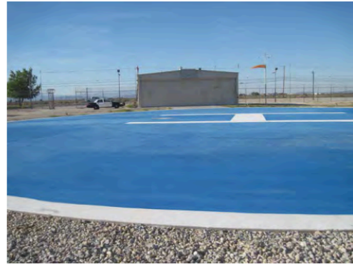
View of Heliport and Aero Hanger (Building 33).
