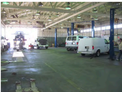
View of hoists in Vehicle Fleet Services Garage.
