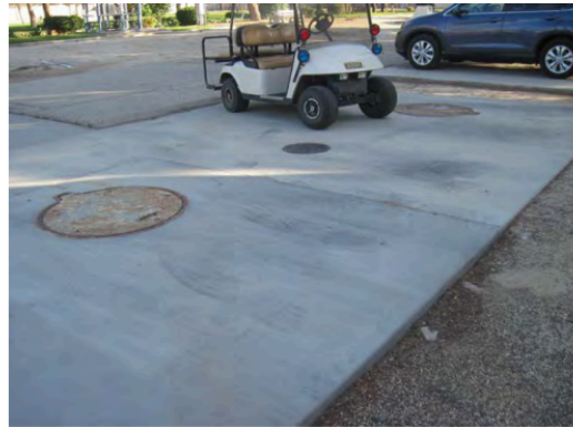
View of 10,000-gallon UST fill port at Steam Plant.
