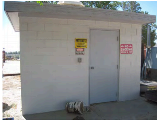
View of Boom Room used to store Hospital hazardous waste.
