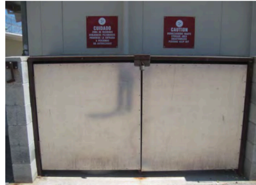
View of biohazardous waste storage container north of Building 2.
