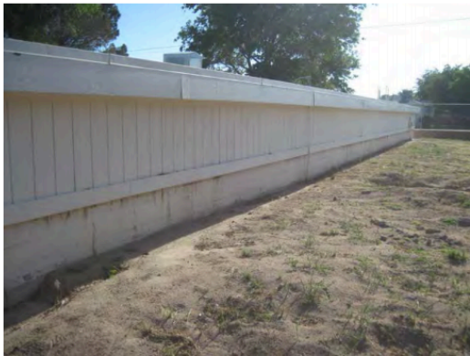
View of 400,000-gallon water reservoir at Mira Loma Detention Facility.
