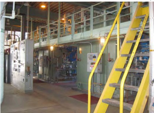
View of Steam Plant.
