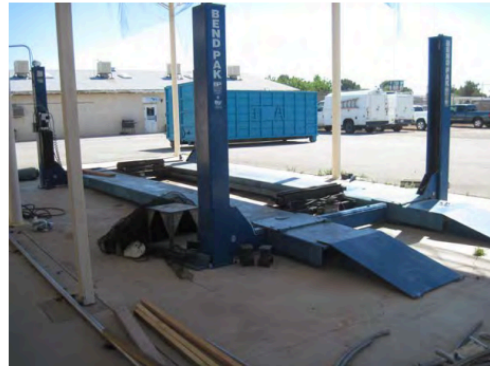
View of hydraulic hoist outside Vehicle Fleet Services Garage.
