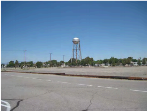
View of 100,000-gallon water tower at Mira Loma Detention Facility.
