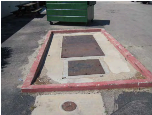
View of clarifier outside Vehicle Fleet Services Garage.
