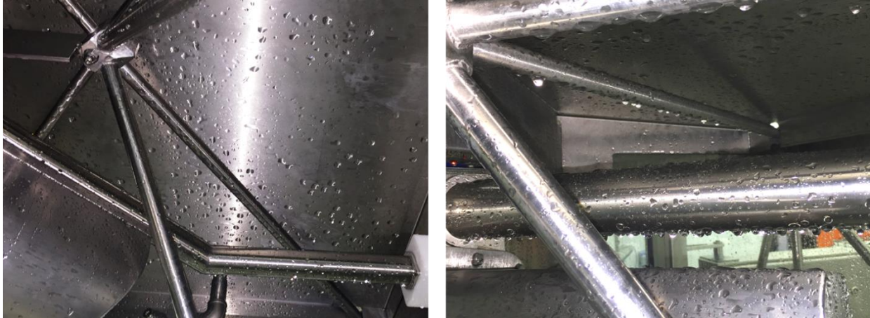
Fig. 51: Improved cleaning behind crossbars in the top area due to the movement of the cleaning device.
