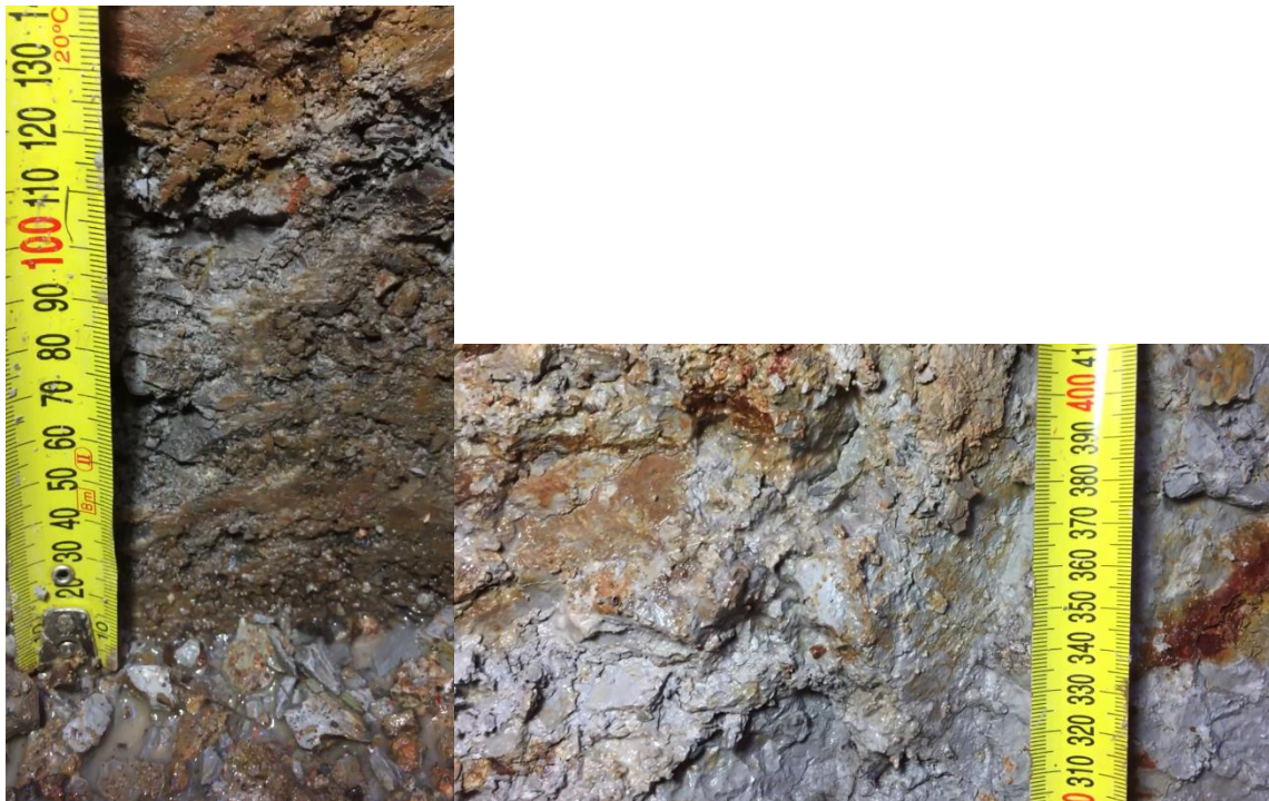
Figure 45. (a) Water accumulated in the base of the completed trench, southern side, western end (video still). Note the position of the measuring tape, with its end resting on the trench base. (b) Clear evidence of water entering the trench approximately 35 cm above the base at the western end (video still, depth ~2.65 m).
