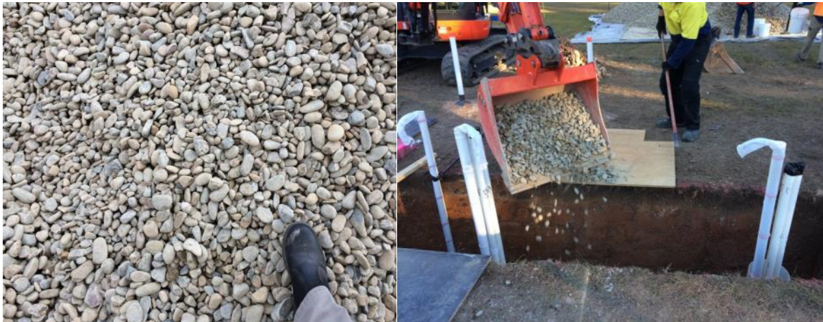
Figure 32. (a) River gravel used to fill the pilot trench. The pebbles were nominally in the range 2 cm to 4 cm in size. (b) Commencement of filling of the trench (Friday 30 th June, 3:30 pm). On Friday the trench was filled to within 1.5 m of the ground surface, at which point it no longer met the definition of a confined space.
