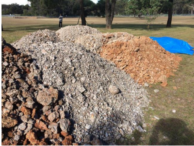
Figure 44. The piles containing material removed from the trench during the excavation, showing differences in coloration of materials from various depths.
