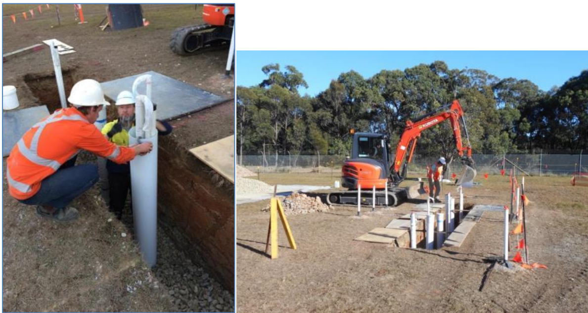
Figure 33. (a) The removal of some PVC pipes which had protected the piezometers when the stones were being emplaced. (b) Final filling of the trench on Tuesday 4 th July. Prior to this time, two additional large diameter sampling experimental tubes (XP1 and XP3) were installed to a depth of ~2 m. See also Figure 50.
