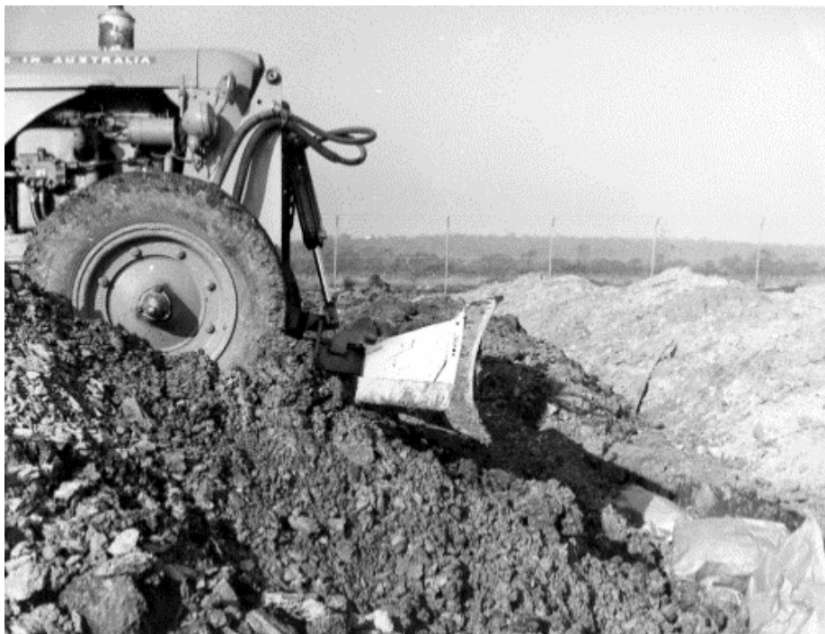
Figure 4. Photograph of soil being pushed into filled trench.
