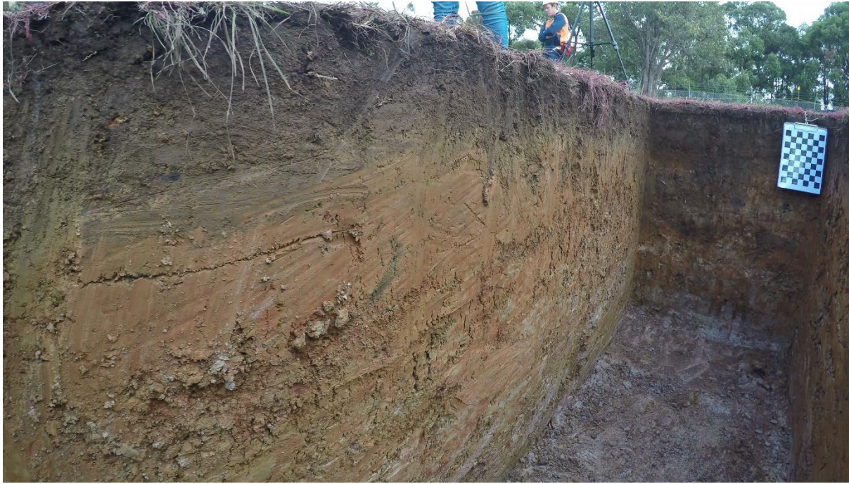
Figure 36. Southern Wall of Pilot Trench.
