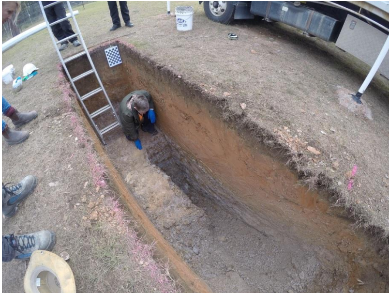
Figure 53. Dr Cath Hughes inspecting seepage into Pilot Trench below the hard shale / siltstone layer at 2.15m depth
