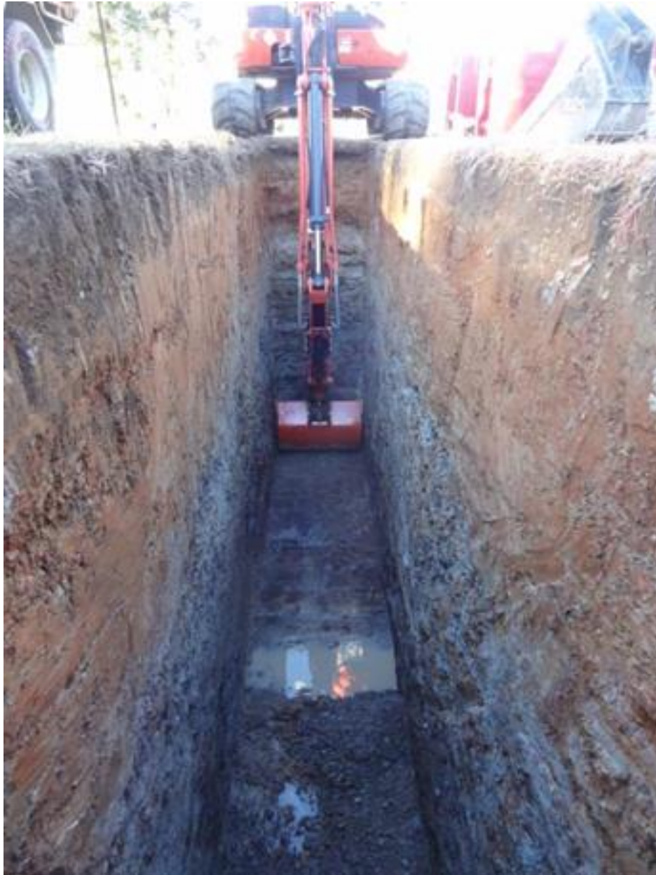
Figure 55. Water accumulating in the trench from the wetter layers observed at depth. The colour gradation in the layers shows a transition from (red) clay to (grey) weathered shale. The boundary occurs between ~0.9 and ~1.1 m.
