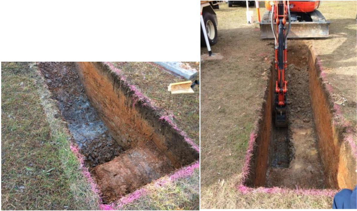
Figure 28. Progress of the trench early on Tuesday 27 th June.
