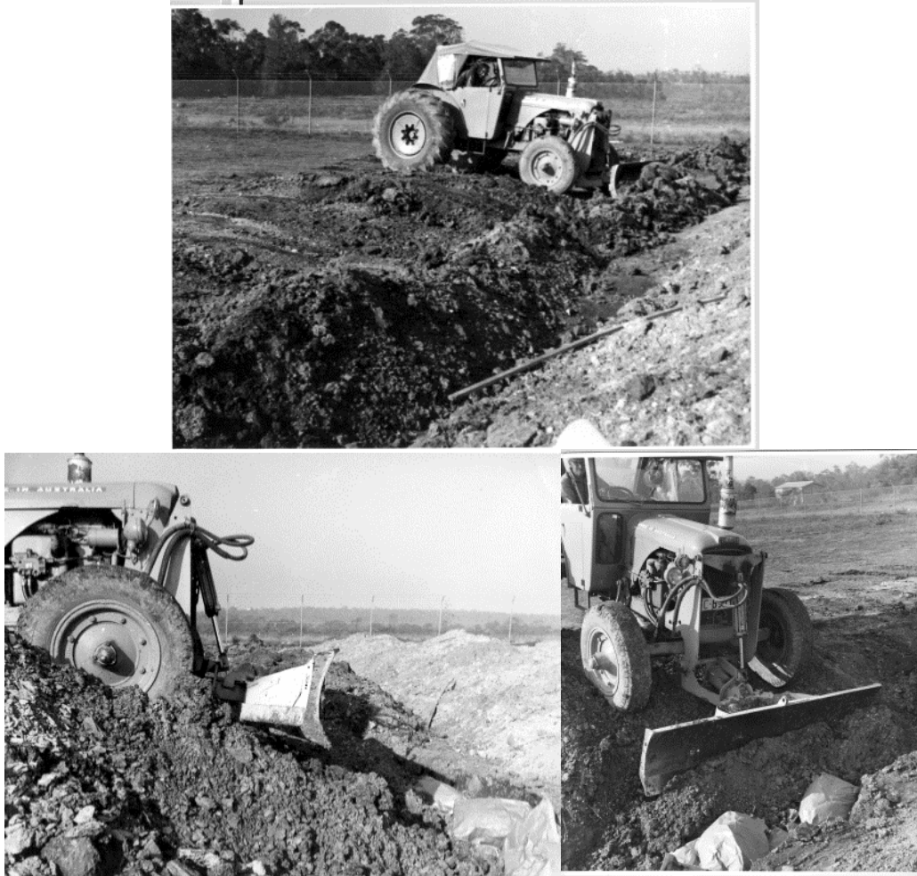
Figure 63. Contemporary photographs covering of disposal trenches. Note the amount of fill materials on the ground surface
