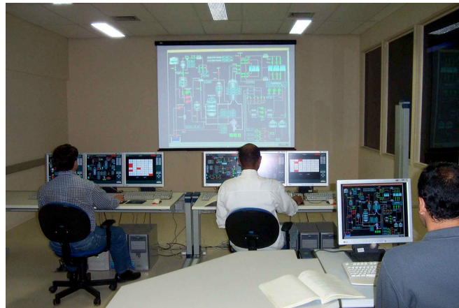
Figure 2. LABIHS advanced control room.
