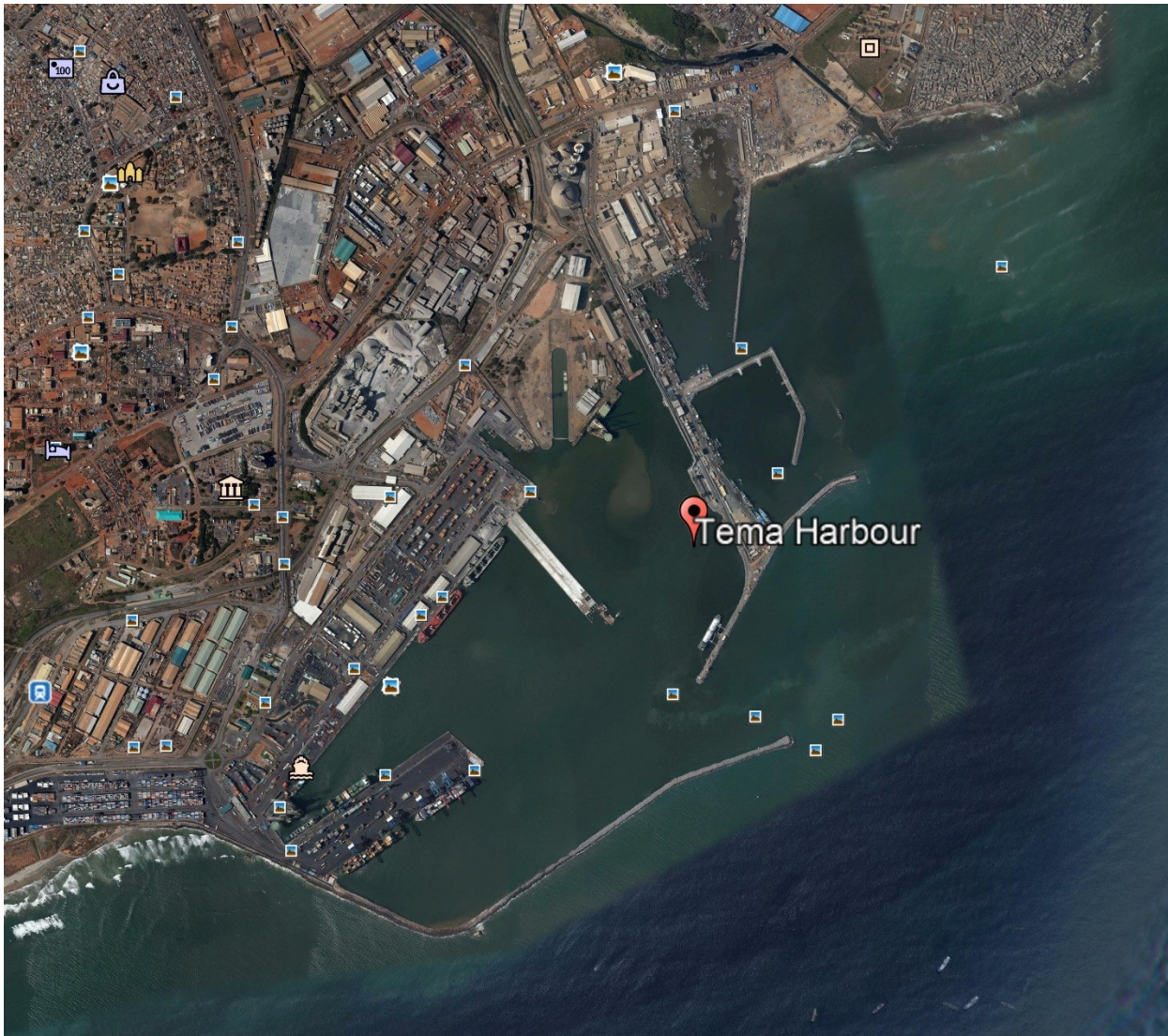
Fig. 1.1 Aerial view of the Tema Harbour (Google Earth)
