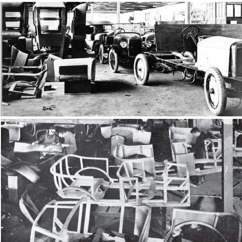
Fig. 6.25 Two views of the T J Richards assembly operation c1922. There was no assembly line and little effort to develop a flow of work in the body building section. SA Library neg B28400/4 & /12
