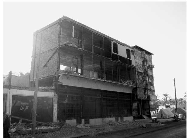
Photo 7. Residence and store building under construction.
