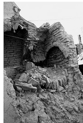
Photo 19. Exceptional seismic damage to adobe house in Kerman City.
