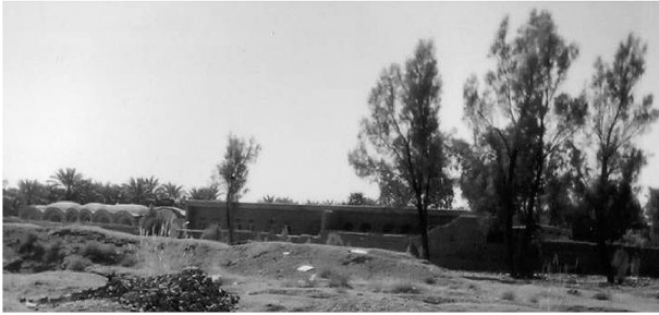
Photo 6. Relatively light damage around site of IIEES array 7.
