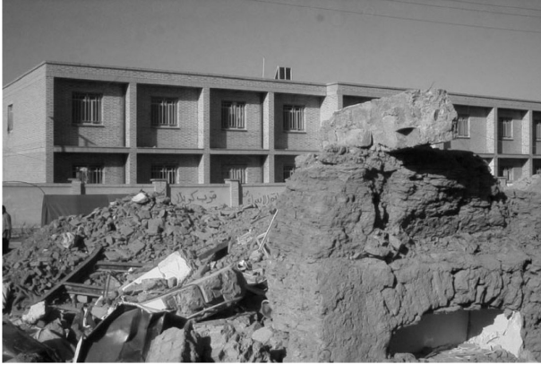
Photo 3. Damaged and undamaged buildings around the site of IIEES array 5.
