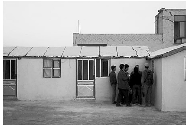
Photo 21. EPS temporary house for evacuation in Bam.
