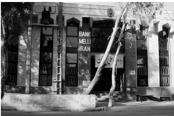
Photo 14. Undamaged bank building in western Bam.
