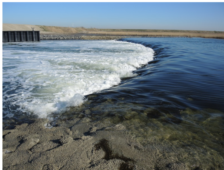
Figure 3 Outflow of saltwater during ebb from the Rammegors (right side of photo) into the Oosterschelde through the culverts in the Krabbenkreekdam (left side of photo). Photo: Tom Ysebaert
