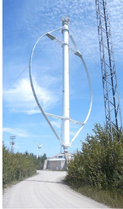
Figure 1.8 : The world tallest vertical axis turbine.
