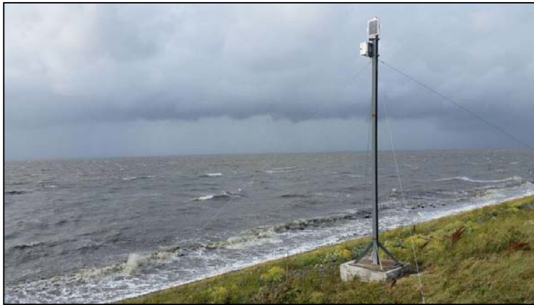
Figure Annex 1-1. Monitoring location Afsluitdijk (photo: Bob Jonge Poerink)
