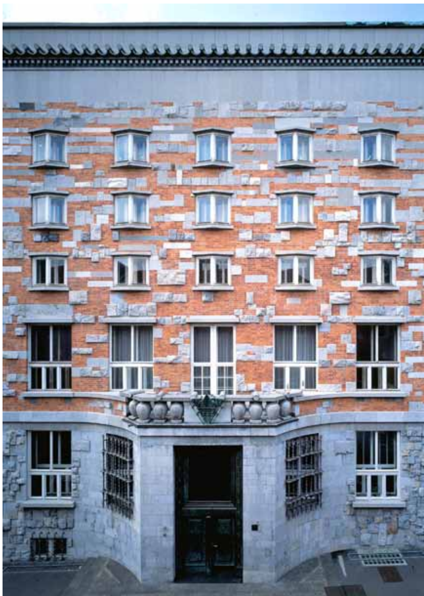
Figure 2. National and University Library, built between 1936–1941 and designed by Slovene architect Jože Plečnik. The front facade was designed as a combination of brick and stone embeddings, some of them archeological remains from the same place. (Photo by Branko Cvetkovič, reproduced with permission of the National and University Library, Ljubljana.)
