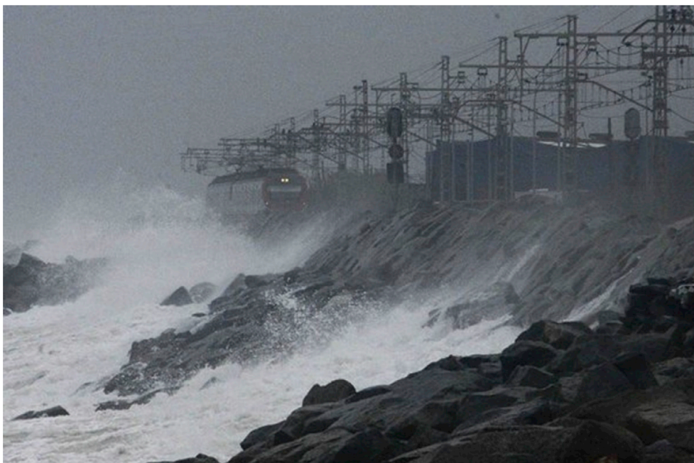
Fig. 5. Affectation of the coastal railway along the Maresme coast during the impact of a storm on March 2003.
