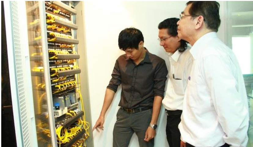
Image 5.2: Server installation process
