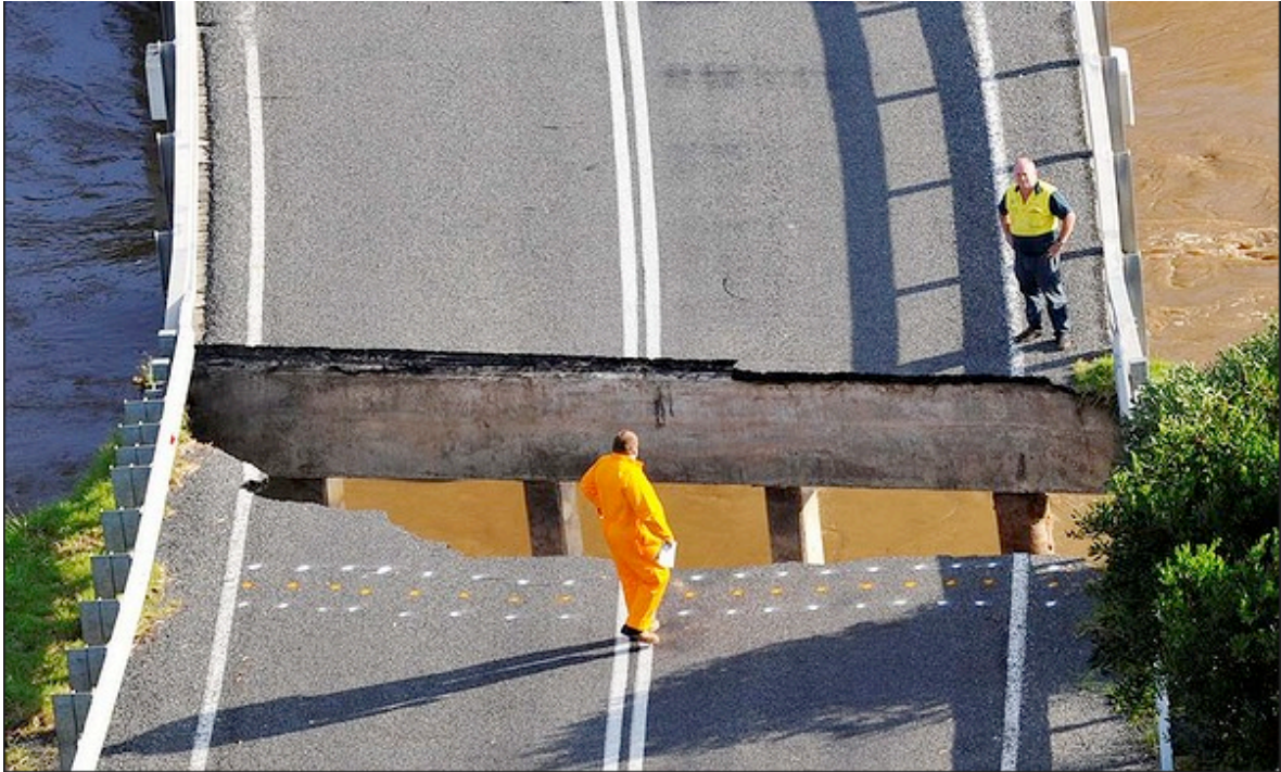
Figure 5.1 – 23 March 2011. Parts of the Darby River Bridge had been completely washed away. Photo: Justin McManus.
