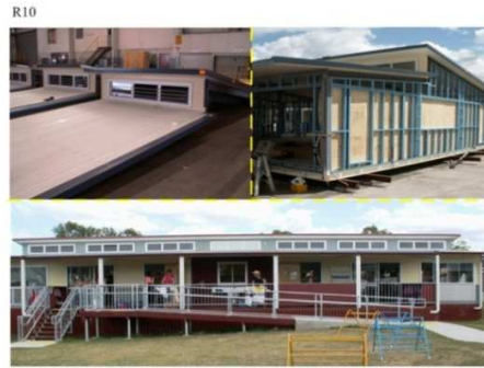
Description: Prefabricated roof systems for offsite built classrooms Source: CRC for Construction Innovation
