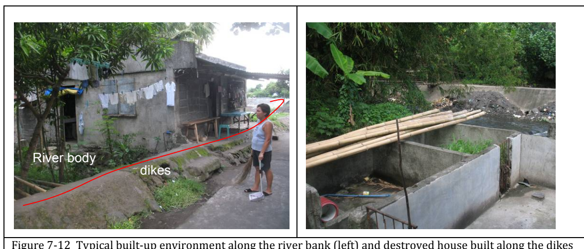
Figure 7-12 Typical built-up environment along the river bank (left) and destroyed house built along the dikes
