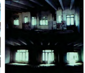
Dagon residence - two views after interior walls' demolition,1994
