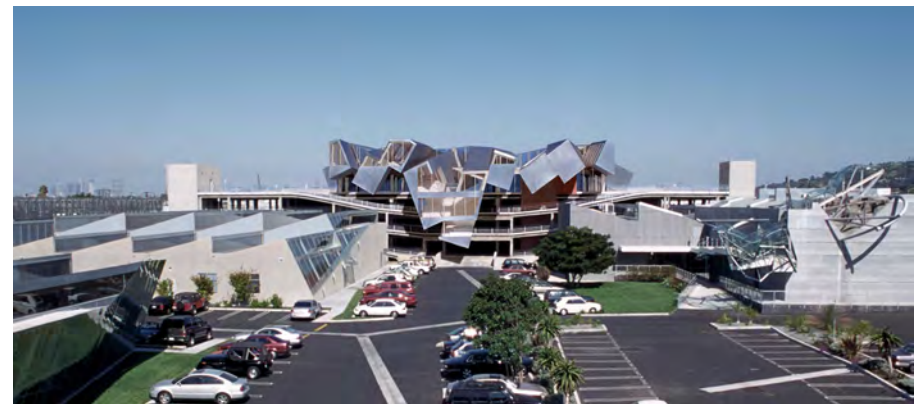
Fig.9 Parking Garage (built) and Pterodactyl (unbuilt) Render, Culver City, California, 1999 -
