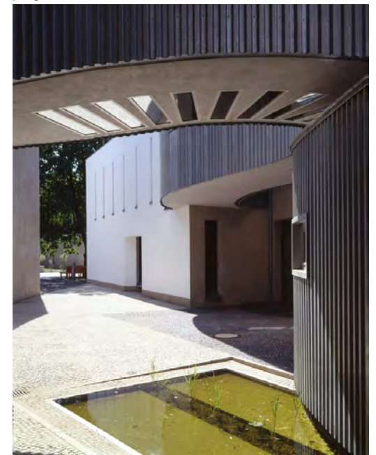
Fig.16 The Heinz Galinski Schule; Jewish Primary School, Ground floor and first floor corridors overlapping each other. Photo, Berlin, 1990-1995
