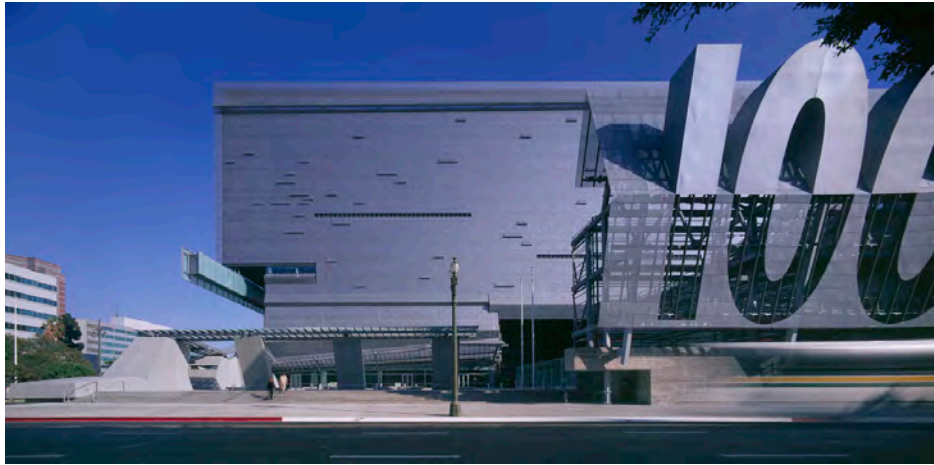
Fig.8 Caltrans District 7 Headquarters, Photo, Roland Halbe LA, 2001-2004
