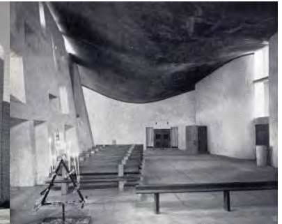
4. Le Corbusier, the chapel of Ronchamp, the floor follows the natural slope, (1950-54)
