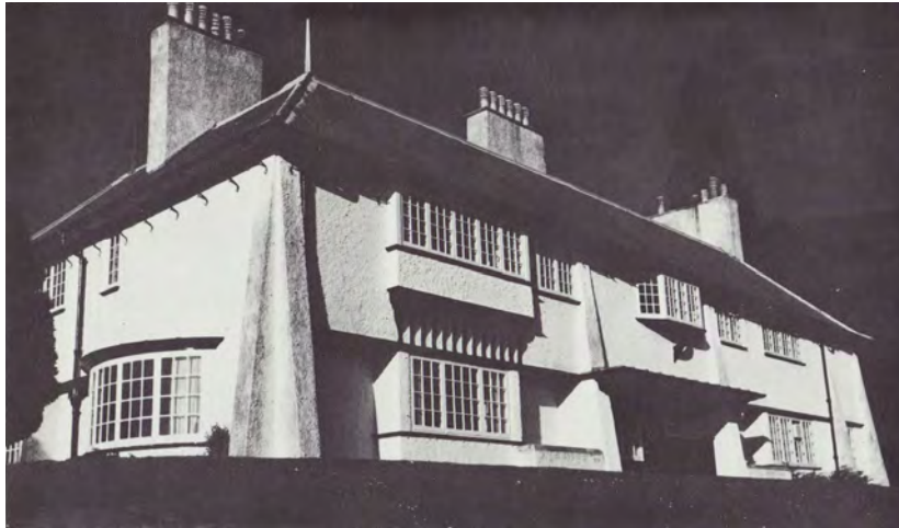
1. Perrycroft, Colwall, Malvern Hills, Herefordshire; garden front from south-west. 1893-1894. Voysey's first large commission. The buttresses rising the full height of the walls, the hipped roof is of green Westmorland slates (a favourite material of Voysey's) penetrated by big, tapering rectangular chimneys.
