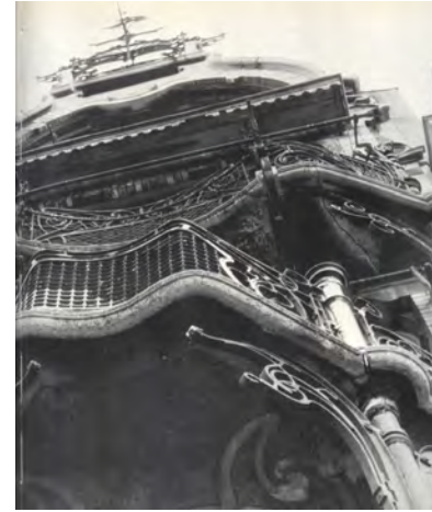
3. Gustave Strouven, Balcony's detail, Residential building, 11 square Ambiorix, Brussels, 1903.
