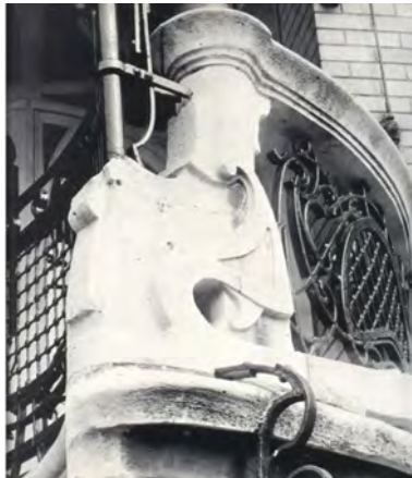
4. Gustave Strouven, Balcony's detail, Residential building, 11 square Ambiorix, Brussels, 1903.
