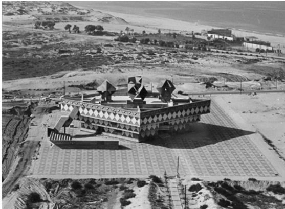
Fig.1 Bat-Yam City Hall built on the vacant land close to the seashore, Overview, Photo, in collaboration Eldar Scharon, Alfred Neumann, Bat-Yam, 1960-63
