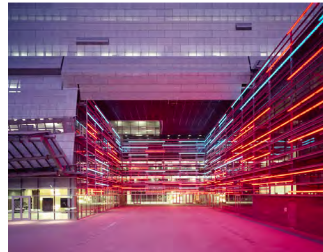
Fig.10 Caltrans District 7 Headquarters, Photo, Roland Halbe, LA, 2001-2004
