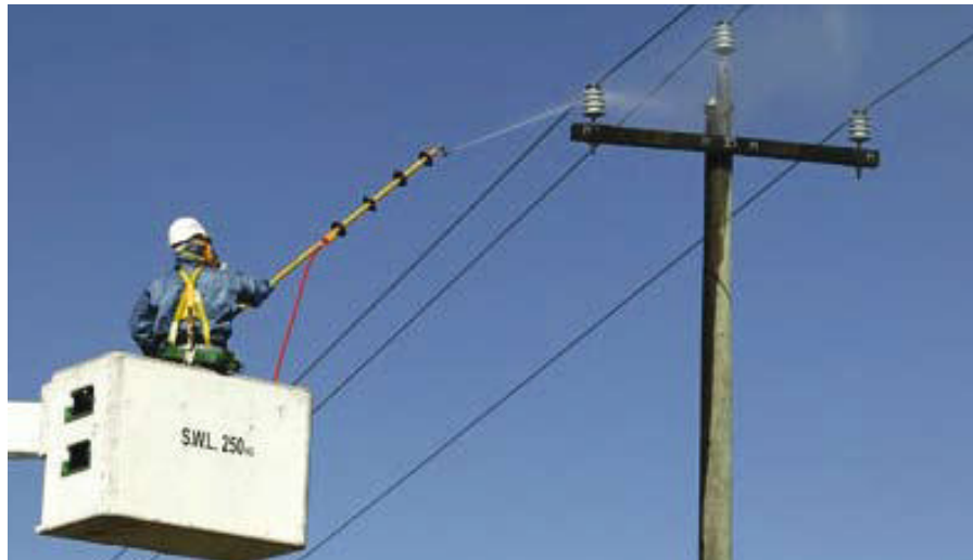
Figure 2.5: Operator spraying silicone compound on pole-top insulators [9]
