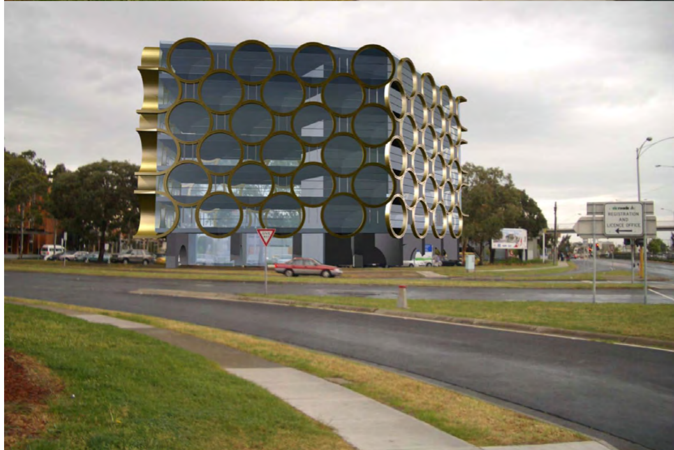
The site from the SE corner – without and with building.
