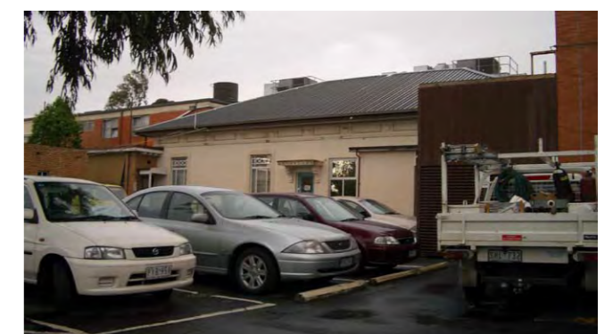
Original Council Offices built 1927 and now service yard
