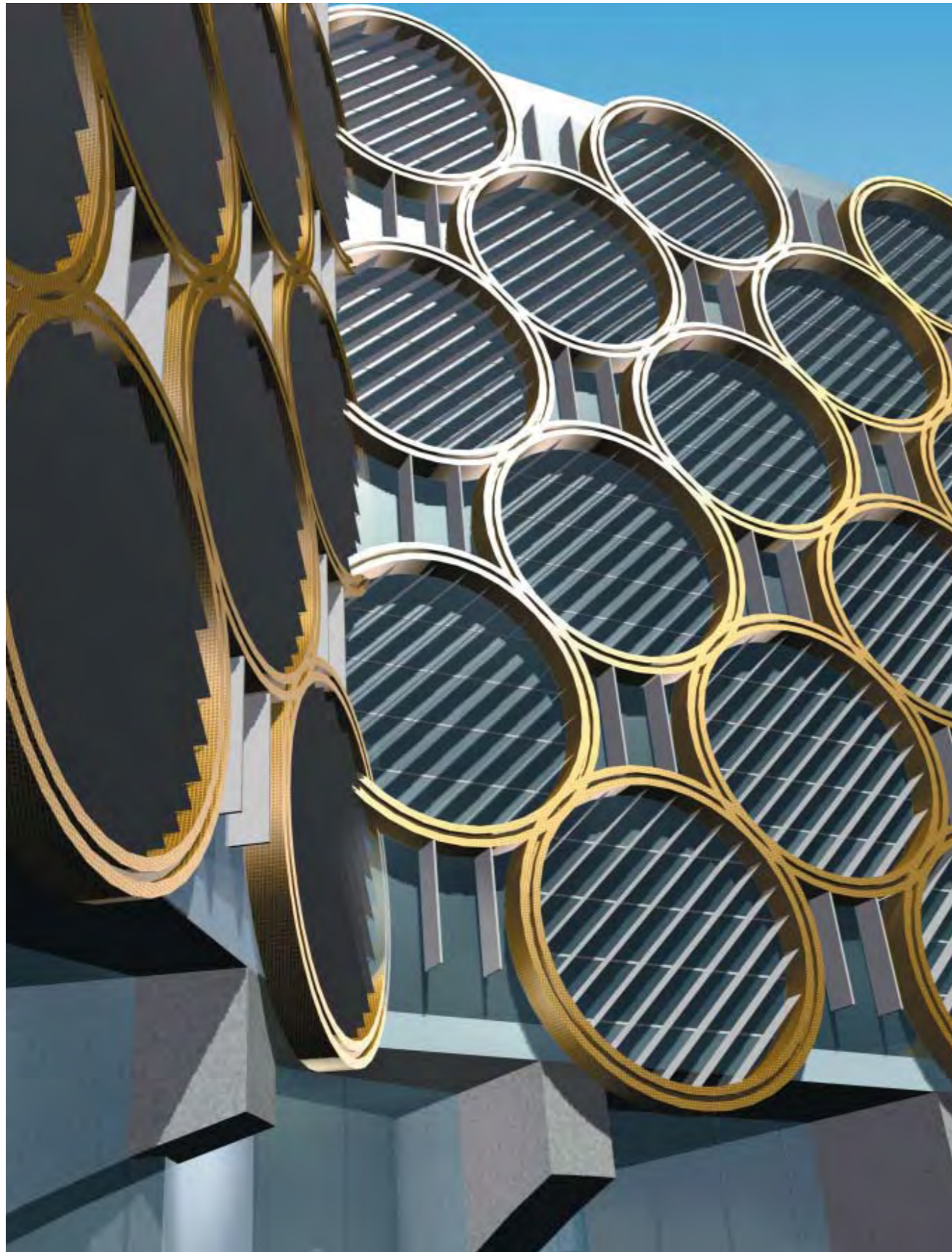
View looking up toward rings from plaza, showing gold mosaic tiles around structurally rings
