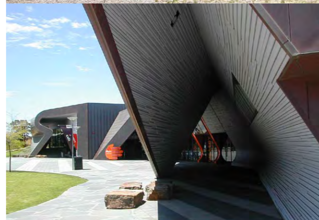
Marion Cultural Centre: 'MAR' letters on front elevation, arcade formed through the 'R' extrusion
