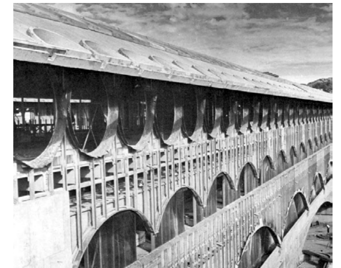
Marin County Civic Center, arches under construction
