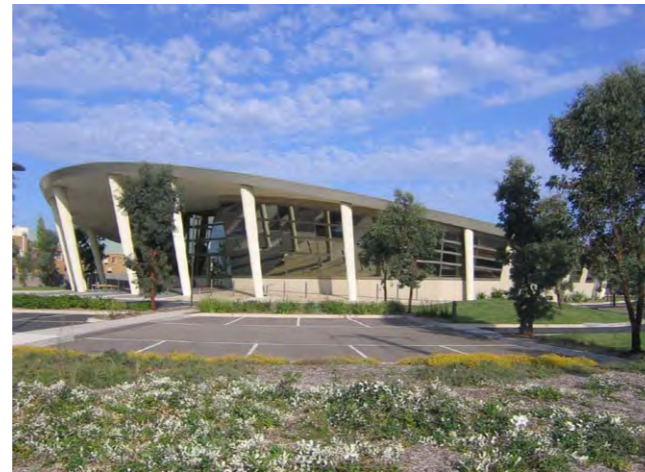
Mill Park Library, Oaten Stanistreet view from road
