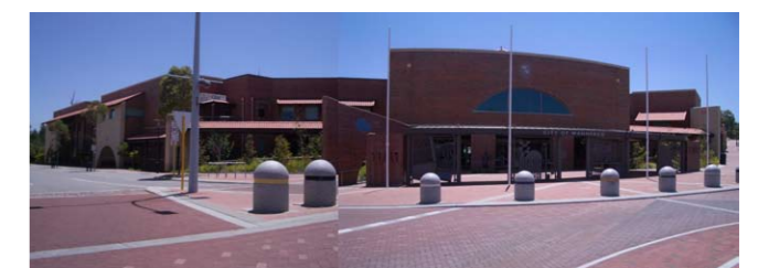
City of Wanneroo Administration Centre & Council Chamber, WA, Woodhead International BDH & Hocking Planning & Architecture, 2000
