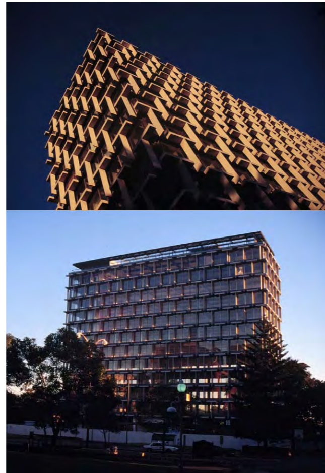
Council House, photographed in 1994 as the being is scheduled and prepared from demolition.
