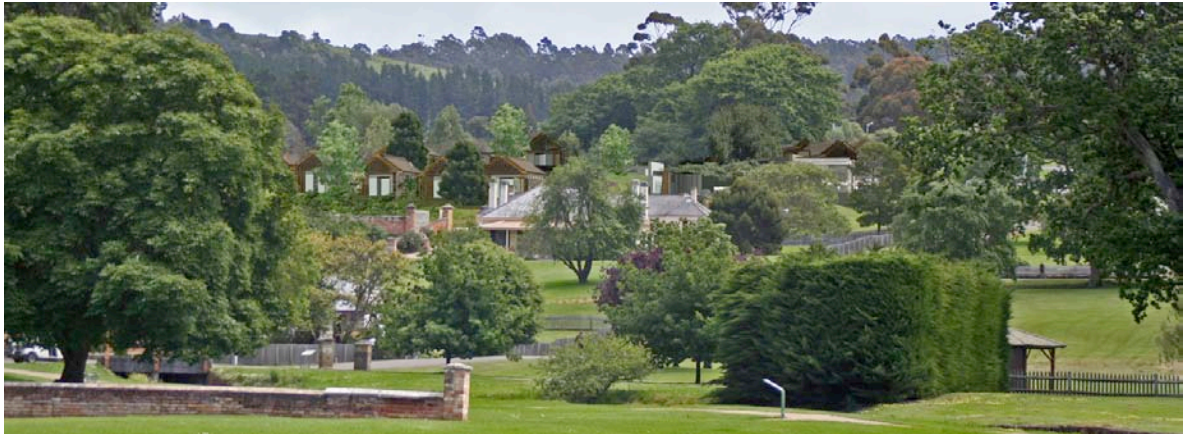
Figure 35: View from main lower part of Port Arthur with the new 'village' in the background
