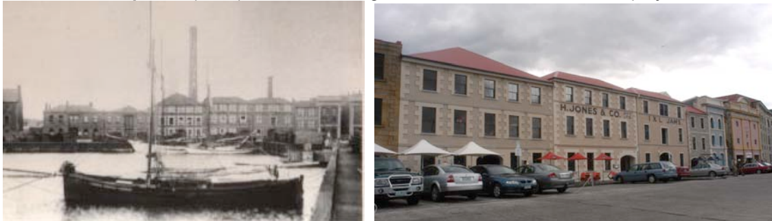
Figures 25/26: IXL Redevelopment: historic view of restored exterior of the warehouses
