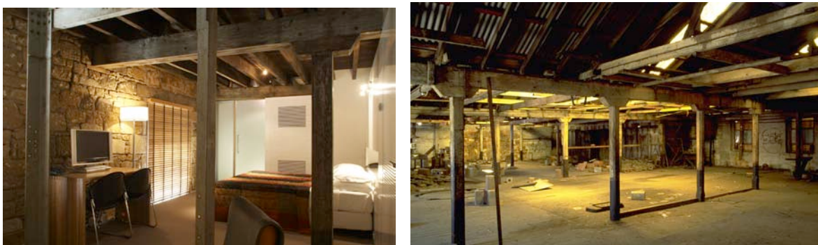
Figures 27/28: IXL Redevelopment: views of finished and unrestored interiors of the warehouses
