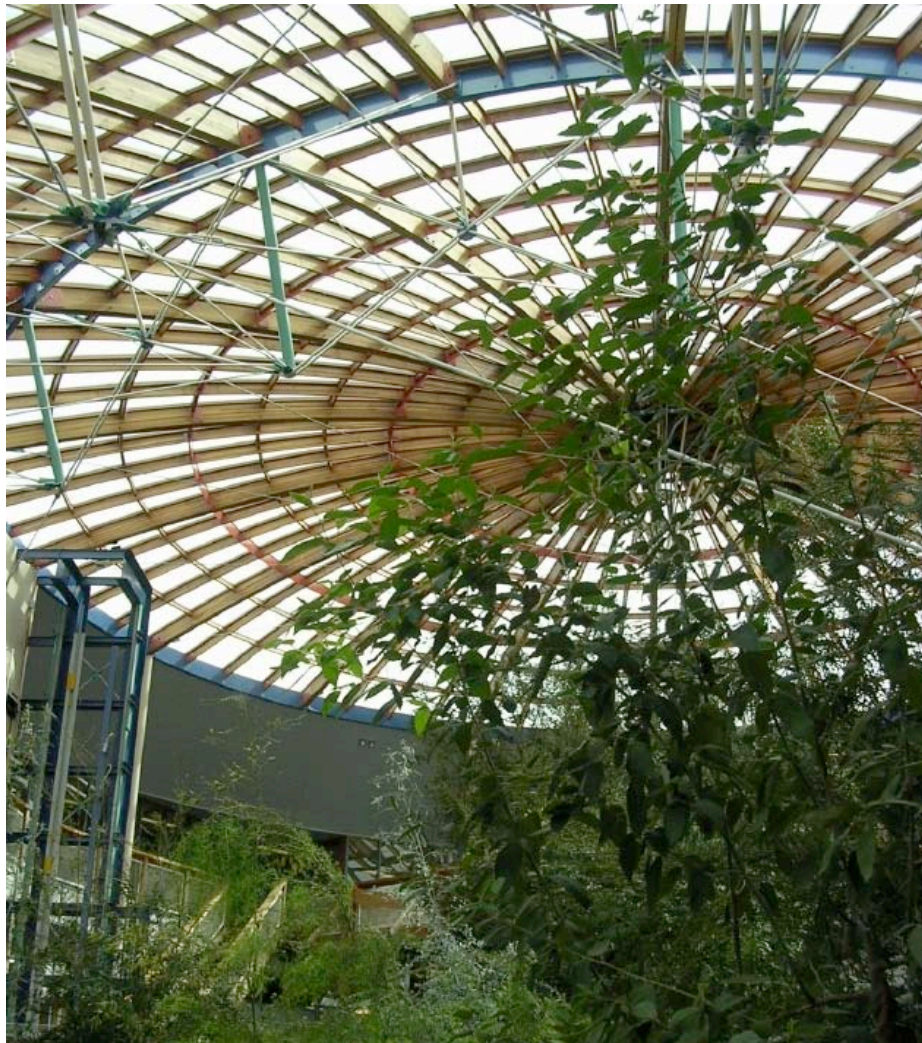
Figure 20: Forestry Headquarters: interior with its landscape
