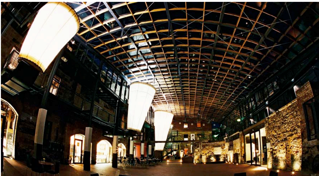
Figure 32: IXL Redevelopment: interior of the glass atrium at night with air chutes doubling as lanterns
