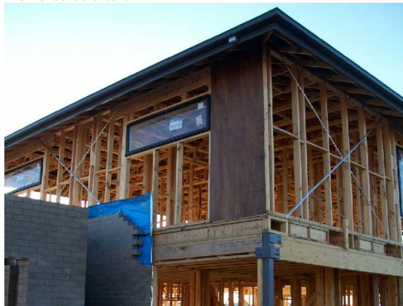
Brick veneer construction
