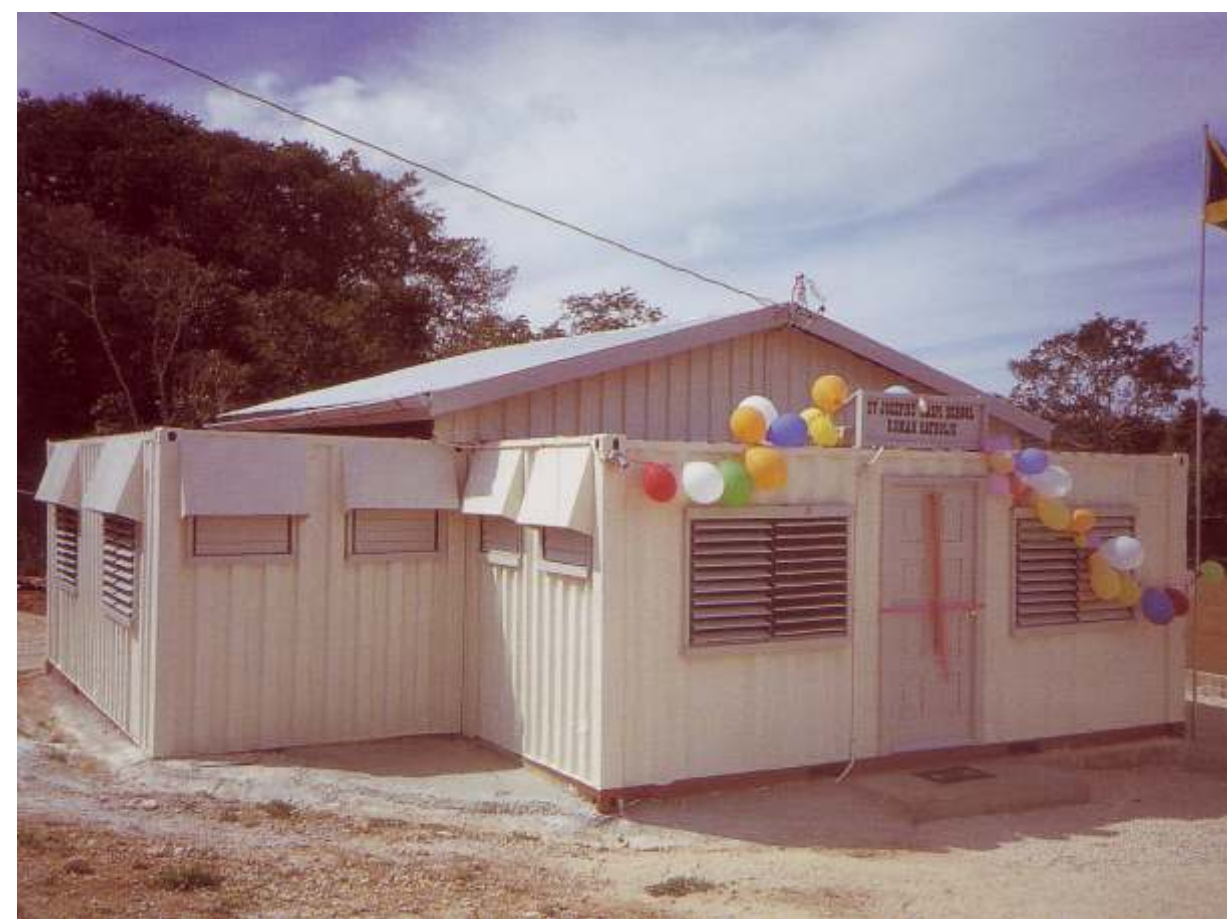
School in Jamaica made from shipping containers(Herbers,2004)
