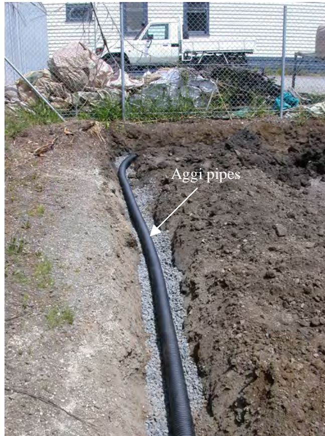
Figure 4.3 Agricultural pipes installed around the car park
