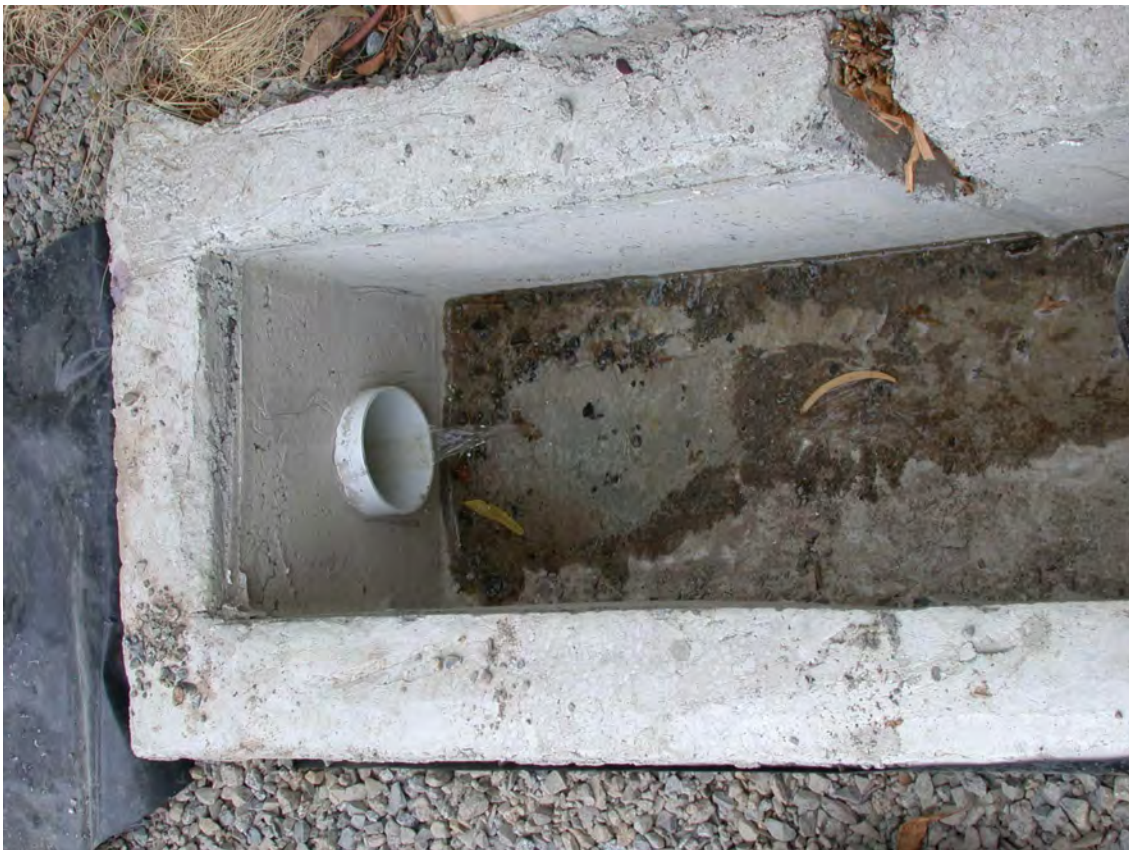
Figure 4.11 Sample Point showing entry of drainage pipe
